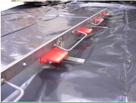
Figure 6-11. Armored joint nosing (Photo courtesy of Canzac and Greenstreak) ( Photo courtesy of PNA Construction Technologies ).
