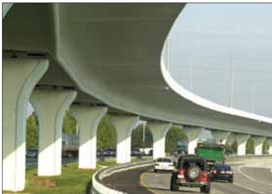
Photo Courtesy of FIGG Bridge Engineers
