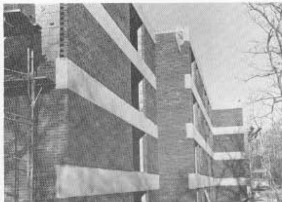
Low-rise apartment building for the elderly combines cast-in-place floors with brick and block walls. It has a two-hour fire-rated floor system.
