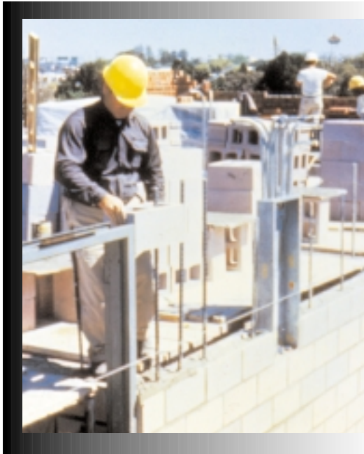
Reinforced concrete masonry wall.
