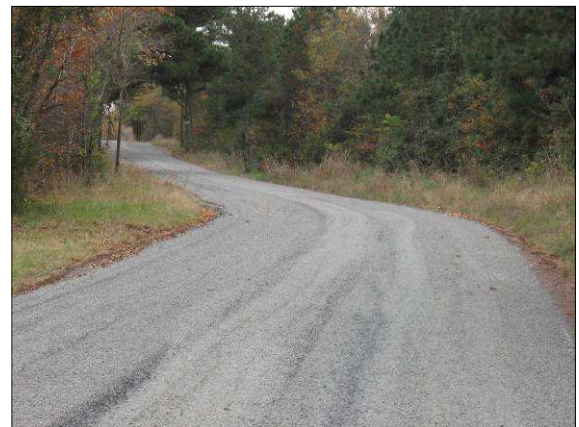
McDuffie Road after the completion of the 2006-2007 Road Improvement Program
