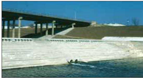
The 4th Low Water Street dam in Texas, USA.
