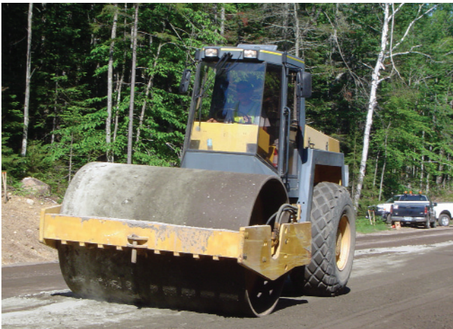
Figure 3.6. Vibratory steel-wheel rollers typically used to compact CTB.
