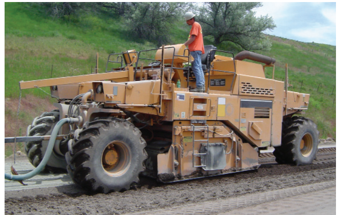
Figure 3.3. Mixing CTB in place using a single-shaft traveling mixer.
