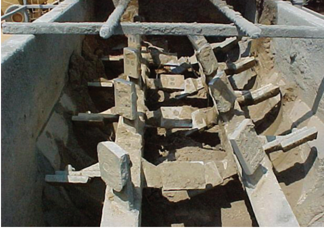
Figure 3.4. Twin-shaft pugmill mixing chamber thoroughly mixes the CTB.
