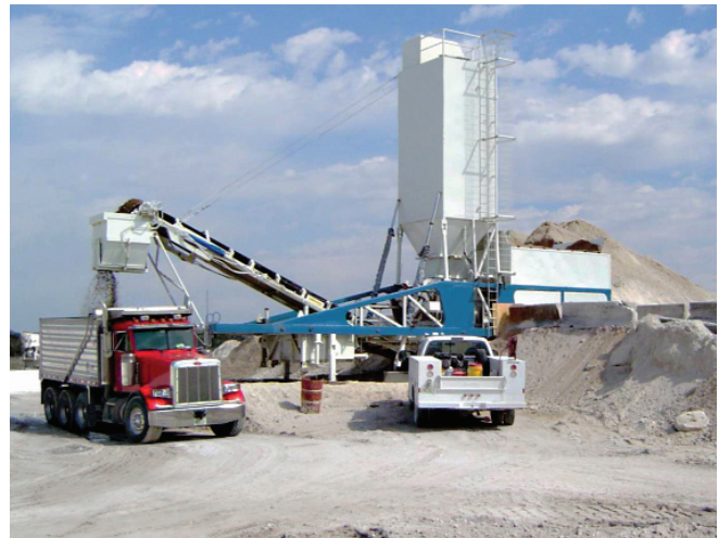
Figure 3.1. Mixing CTB in a continuous-flow-type pugmill.
