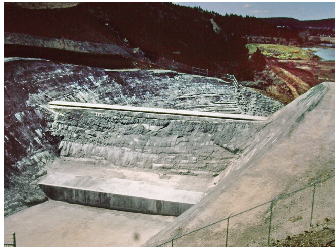
FIGURE 2-8. Outlet channel protection (Ochocho Dam, OR).
