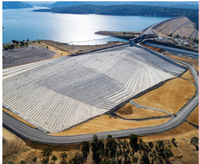
FIGURE 1-12. Auxiliary spillway control section (Oroville Dam, CA).
