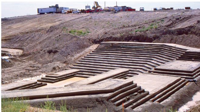
FIGURE 1-14. RCC drop structure in outlet channel (Standley Lake Dam, CO).
