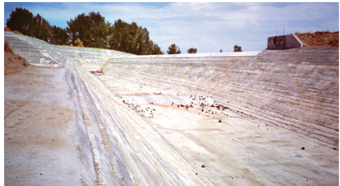
FIGURE 1-15. Erosion protection (Cold Springs Dam, OR).
