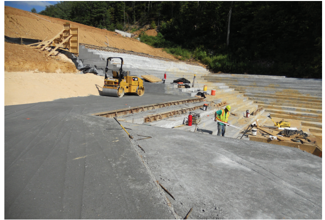
FIGURE 9-31. Placement of RCC at transition area.
