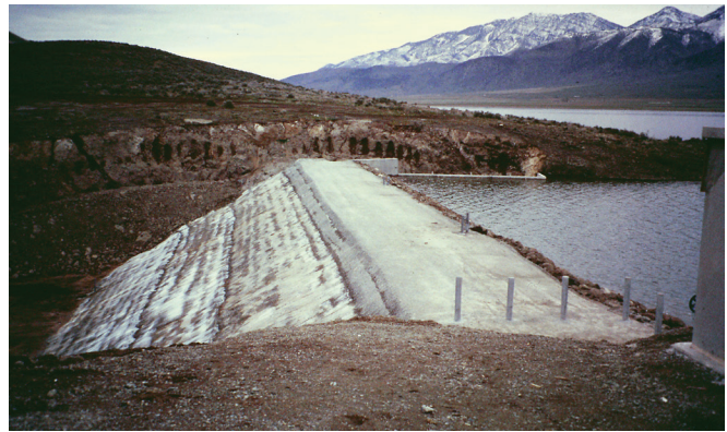
FIGURE 6-8. Compacted, unformed RCC downstream face (Mona Dam, UT).
