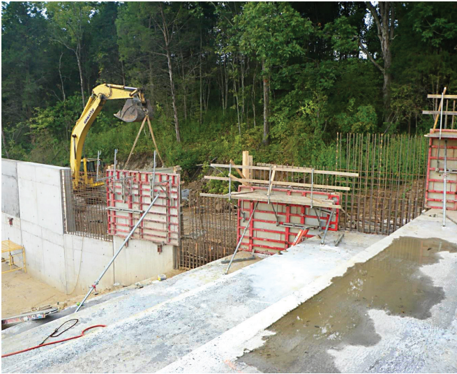
FIGURE 6-48. Conventional concrete training wall construction (Stoney Creek Dam, VA).
