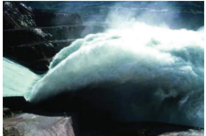
FIGURE 1-1. Spillway flow in RCC repair area (Tarbela Dam, Pakistan).
