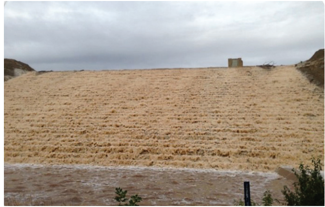
FIGURE 10-5. Overtopping spillway activated during storm event (Left Hand Dam, CO).
