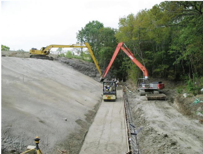
FIGURE 9-7. RCC delivery with long stick hydraulic excavators.
