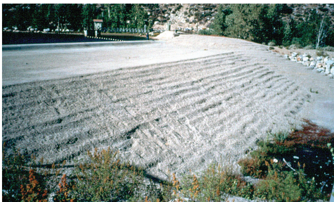
FIGURE 6-7. Uncompacted, unformed RCC downstream face (Bishop Creek Dam No.2, CA).
