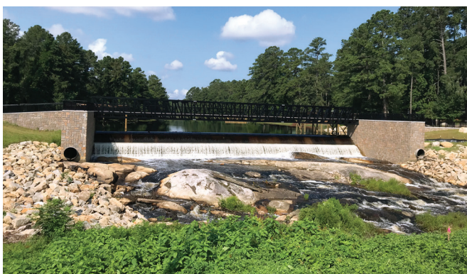
FIGURE 6-14B. Formed liners used to simulate appearance of stone masonry (Gibson Pond Dam, SC).
