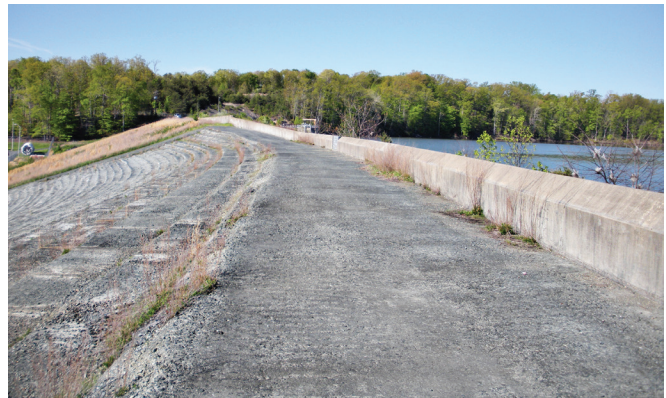
FIGURE 6-19. Sharp crested weir (Smith Lake Dam, VA).
