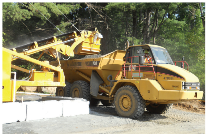
FIGURE 9-5. Haul truck being loaded with fresh RCC at mixing plant.
