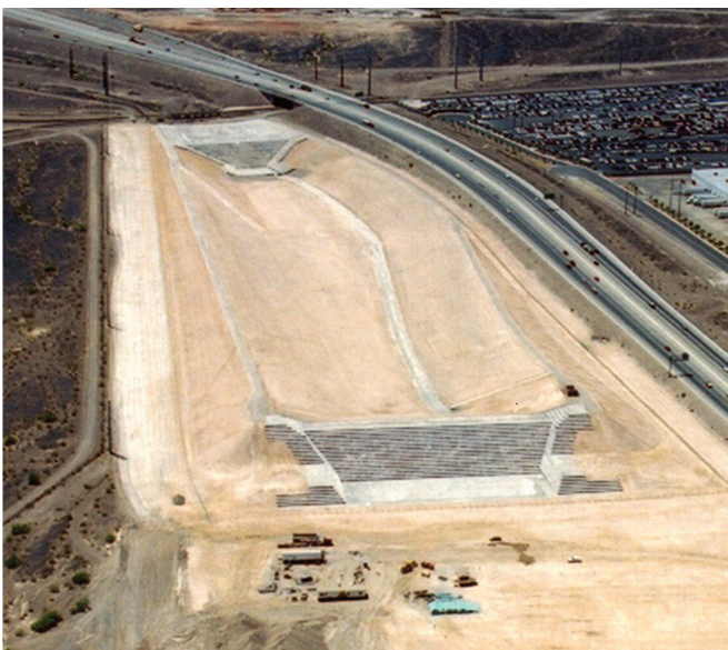
FIGURE 1-11. Pioneer Detention Basin, NV.
