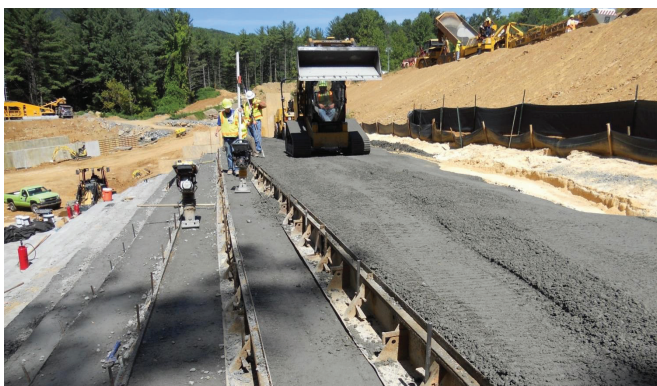
FIGURE 6-14A. Formed RCC steps, 1-ft high (Stoney Creek Dam, VA).
