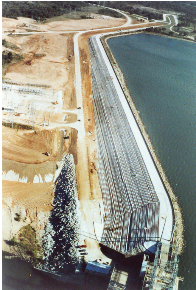
FIGURE 1-7. Alvin J. Wirtz Dam, TX.
