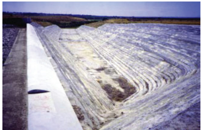
FIGURE 2-9. RCC side channel spillway (Cold Springs Dam, OR).
