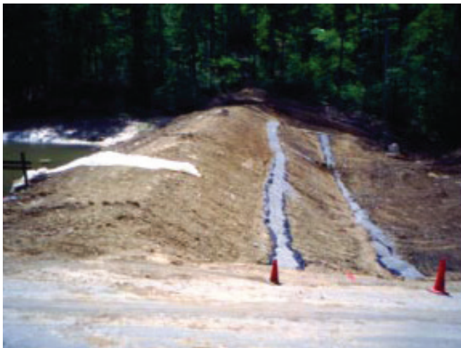
FIGURE 6-37. Trench drain construction prior to RCC placement (McBride Dam, OH).
