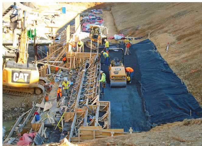
FIGURE 9-13. Hand placement of RCC.
