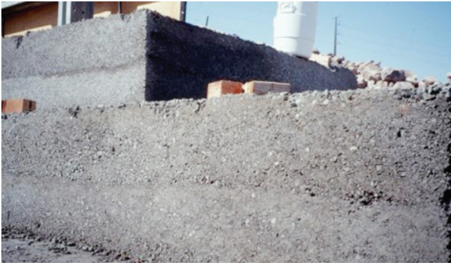
FIGURE 9-21. Good RCC face.
