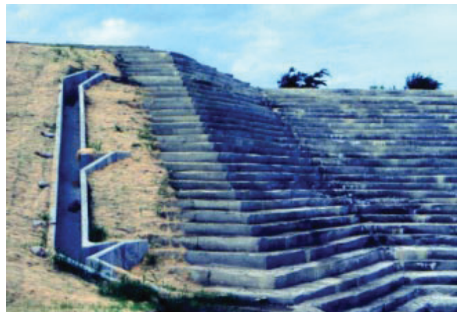
FIGURE 6-40. Concrete drain outlet structure (South Prong Dam, TX).
