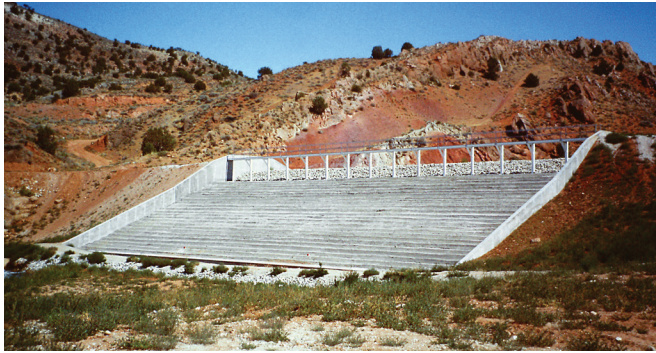
FIGURE 6-23. Fuse plug (Gunnison Dam, UT).
