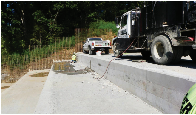
FIGURE 6-13. Formed grout enriched RCC steps.
