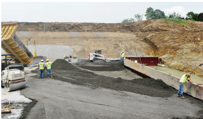
FIGURE 9-15. Formwork layout performed by licensed surveyor to control lift geometry.
