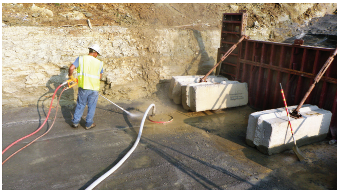
FIGURE 9-28. Preparation of cold joint.
