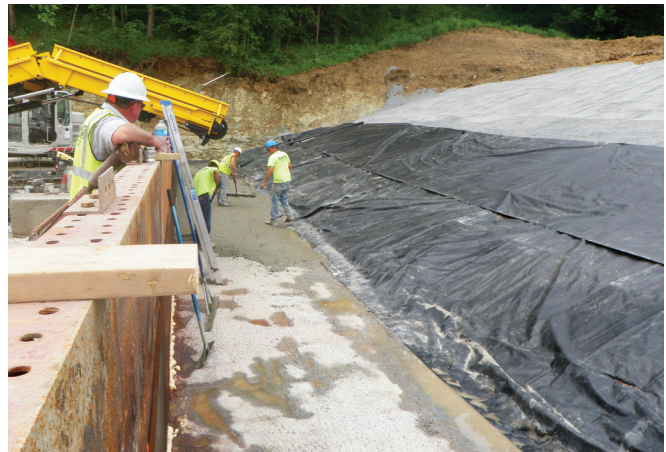
FIGURE 9-30. Bedding mortar placement.
