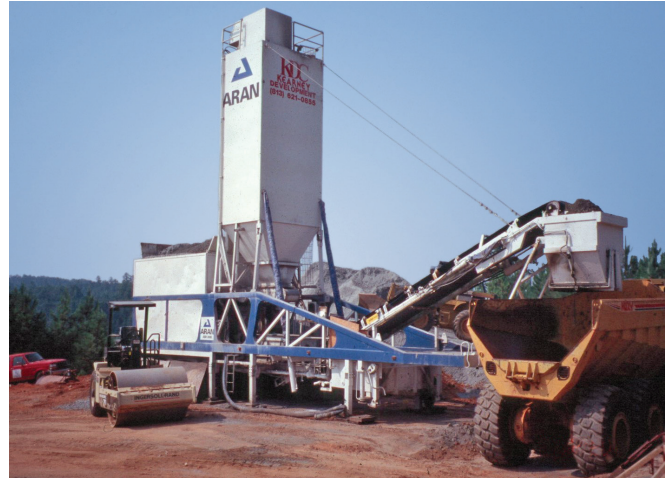
FIGURE 9-3. Continuous mix plant.
