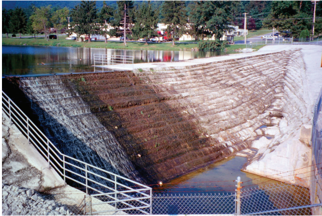
FIGURE 2-3. RCC service spillway (Lower Lake Royer Dam, MD).
