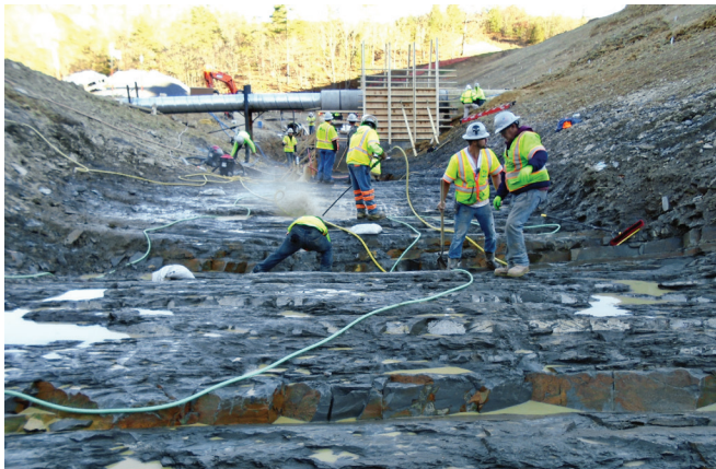
FIGURE 9-2. Foundation preparation and cleaning using compressed air with water.
