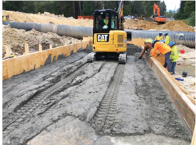
FIGURE 7-3. Typical fresh IVRCC surface.
