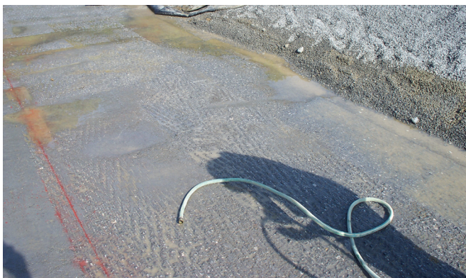
FIGURE 9-29. Roughened surface prepared using skid-steer mounted grinding tool.
