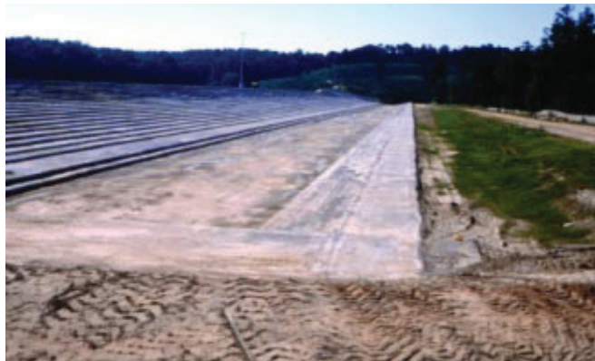
FIGURE 6-28. Stilling basin constructed of RCC (Lake Tholocco Dam, AL).
