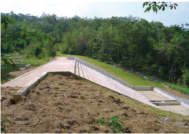
FIGURE 6-16. Broad crested weir (Great Gorge Dam, NJ).
