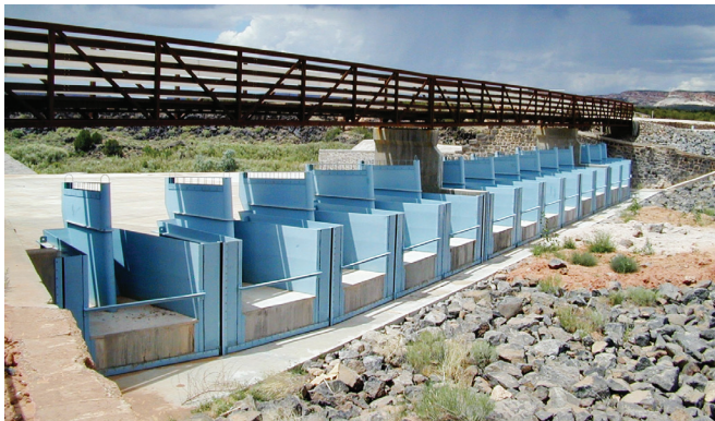
FIGURE 6-24. Fuse gates (Black Rock Dam, NM).
