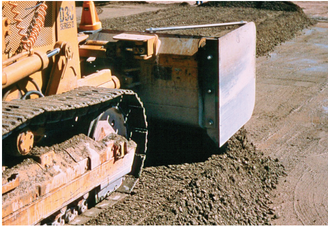
FIGURE 9-14. Modified bulldozer blade to minimize segregation of RCC.
