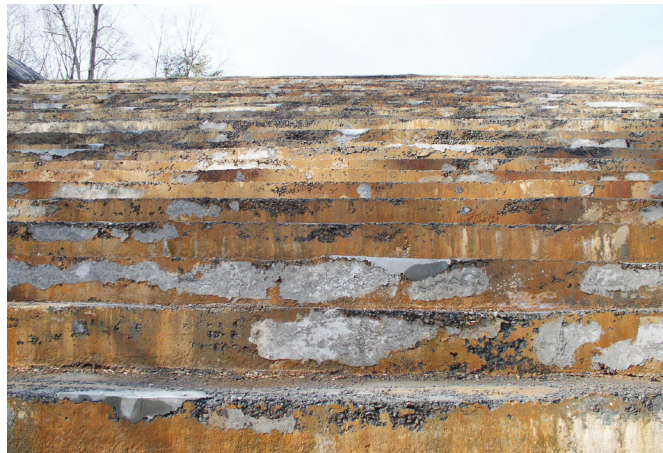
FIGURE 9-32. Results of inadequate effort to patch substandard RCC surface.
