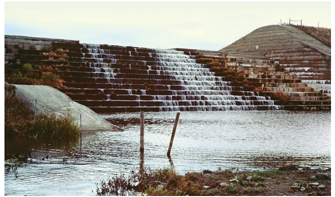
FIGURE 2-5. Combined principal and auxiliary spillway (Ponca Dam, SD).
