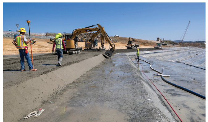
FIGURE 2-6. Armored earthen spillway (Oroville Dam, CA).
