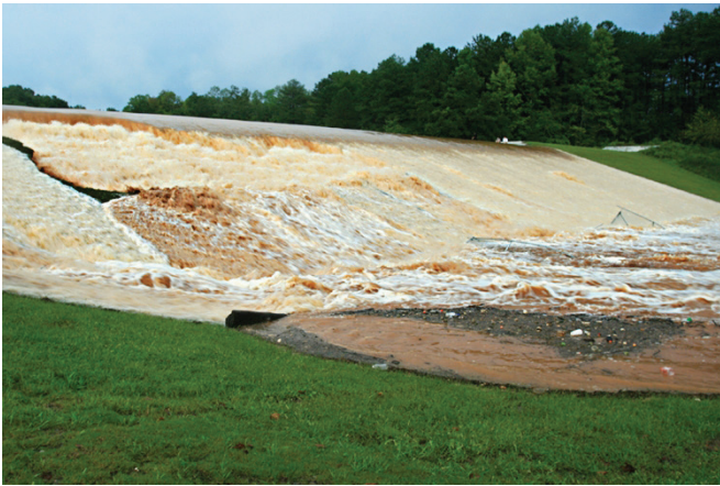
FIGURE 10-3. Overtopping spillway during 2009 flood (Yellow River Structure Y-16, GA).
