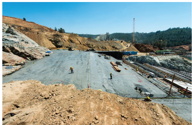
FIGURE 1-13. Foundation support (Oroville Dam, CA).
