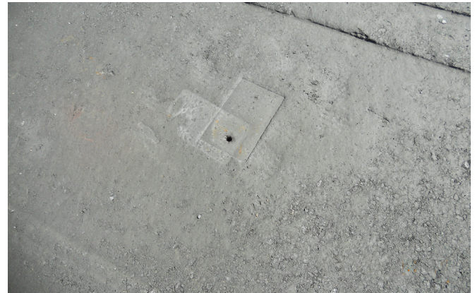
FIGURE 9-18. Typical good-quality RCC surface texture.
