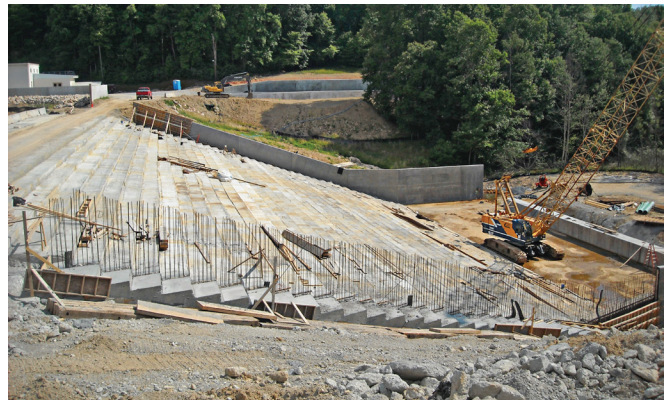
FIGURE 6-45. Conventional concrete training walls on completed RCC (Bear Creek Dam, VA).
