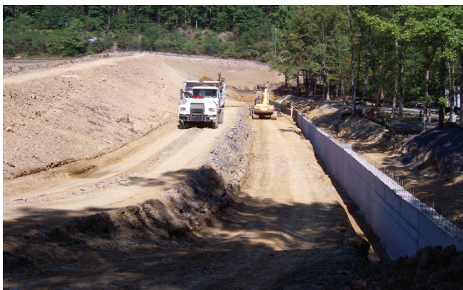
FIGURE 6-31. Downstream cutoff wall (Poe Valley Dam, PA).
