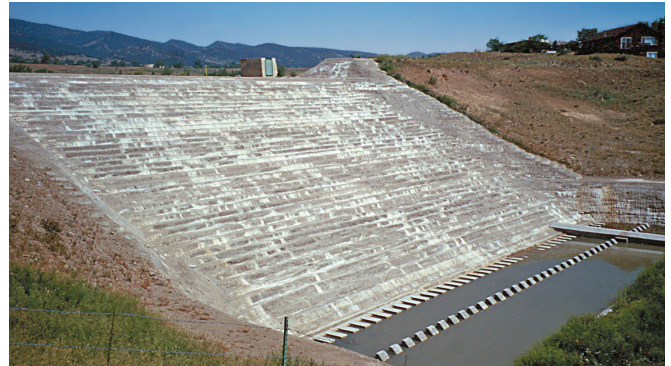
FIGURE 9-20. Unformed, compacted RCC steps.
