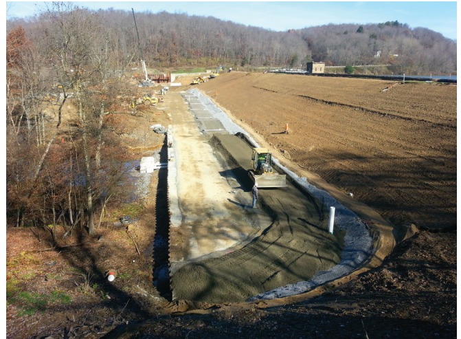
FIGURE 6-38. Blanket drain construction during RCC placement (Lake Oneida, PA).
