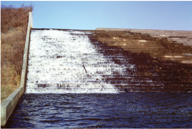
FIGURE 2-1. Principal spillway (Butler Dam, GA).
