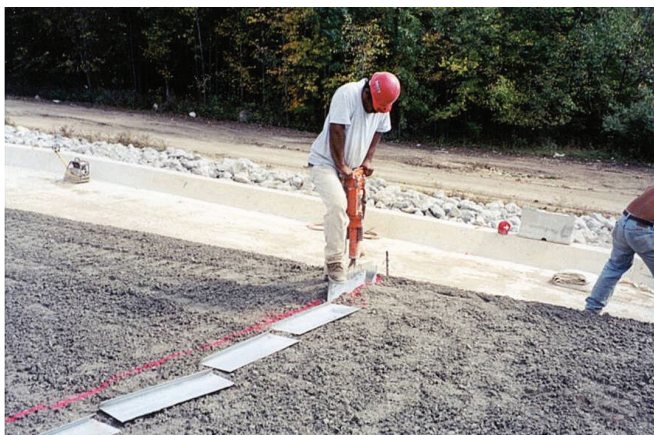
FIGURE 9-26. Steel plate inserted into fresh RCC to create control joint.
