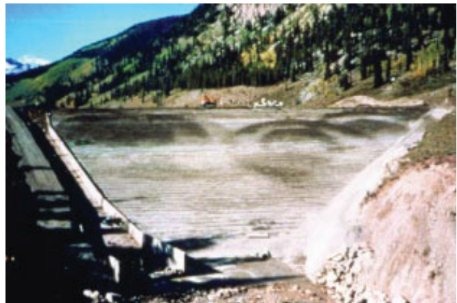
FIGURE 1-6. Spring Creek Dam, CO.
