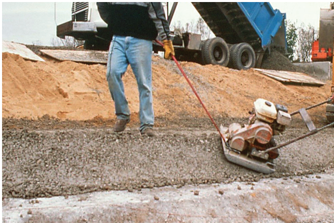
FIGURE 9-16. Vibratory plate compactor used to compact unformed RCC steps.
