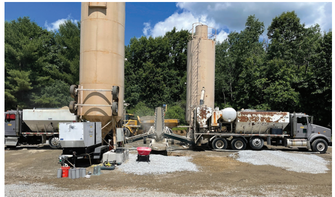
FIGURE 9-4. Mobile volumetric concrete mixer trucks being used to produce RCC.
