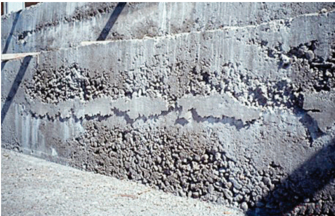
FIGURE 9-22. Fair RCC face.
