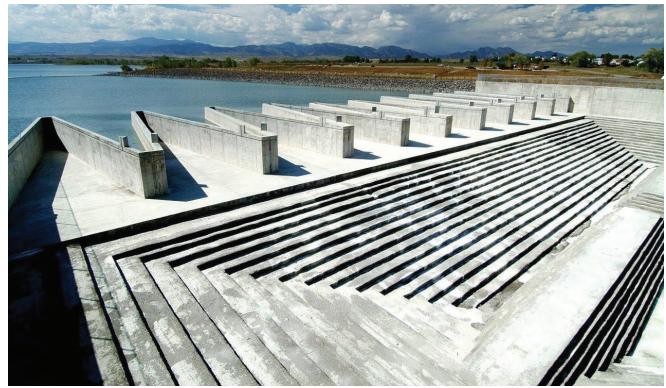
FIGURE 6-18. Labyrinth crest weir (Standley Lake Dam, CO).
