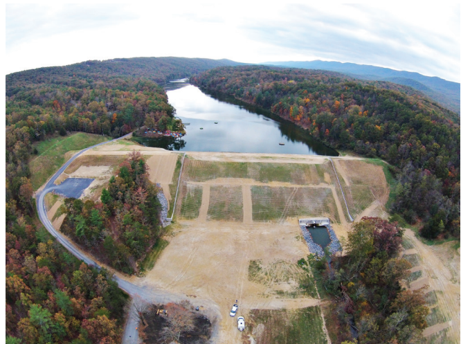
FIGURE 6-49B. RCC spillway after topsoil cover is placed (Lake Laura Dam, VA).
