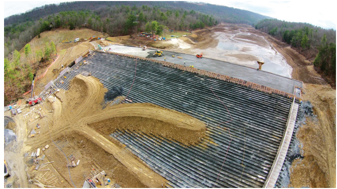
FIGURE 6-49A. RCC spillway before topsoil cover is placed (Lake Laura Dam, VA).
