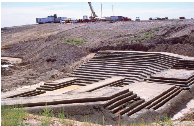
FIGURE 2-7. Outlet channel protection (Standley Lake Dam, CO).
