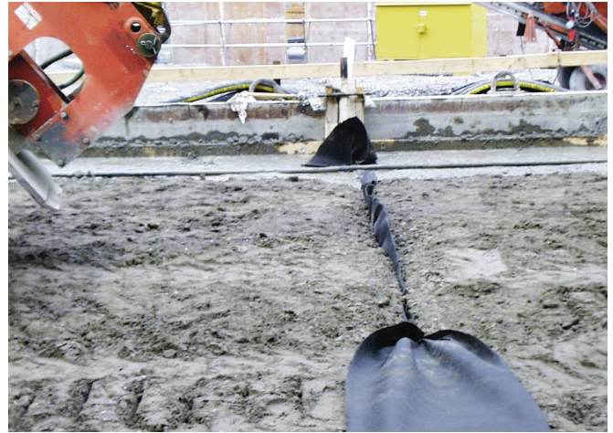
FIGURE 9-27. Plastic sheeting buried in RCC to create control joint.
