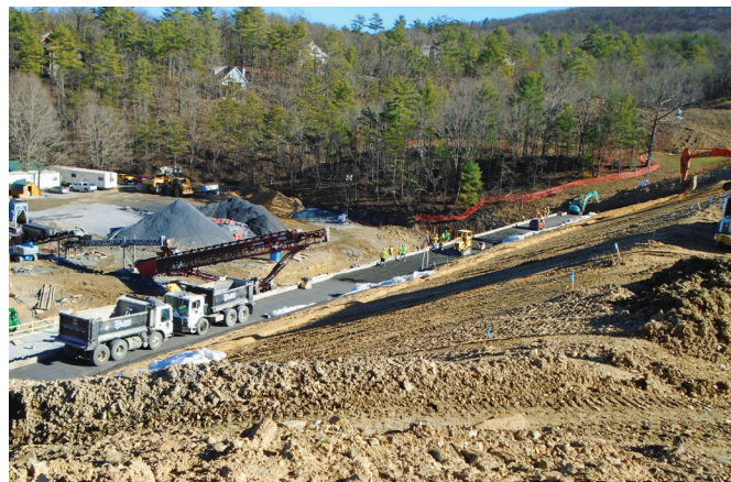
FIGURE 9-12. Typical RCC spreading and compaction sequence at placement area.
