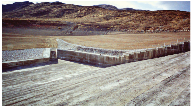
FIGURE 6-44. Vertically formed RCC training walls (Red Rock Canyon Detention Dam, NV).
