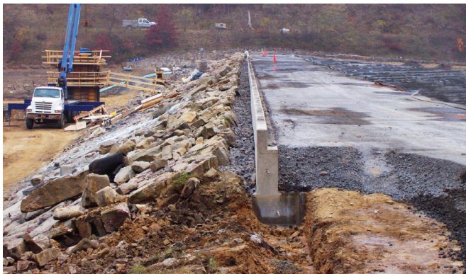
FIGURE 6-30. Upstream cutoff wall (Poe Valley Dam, PA).
