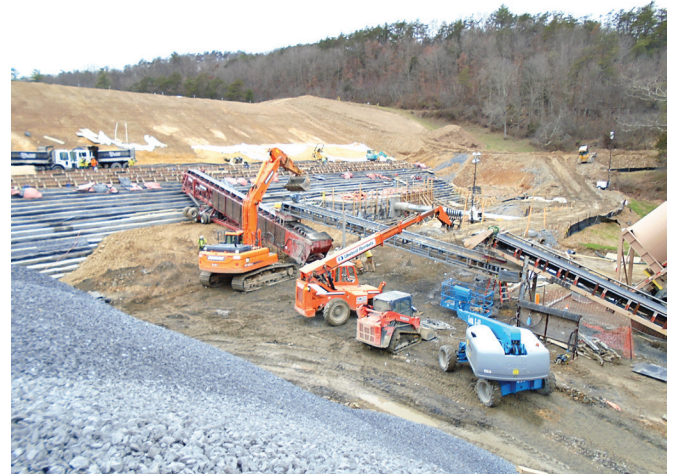
FIGURE 9-8. RCC moved to placement area using conveyor delivery system.
