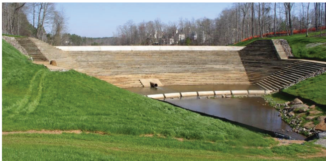
FIGURE 6-41. Formed slope RCC training walls (Yellow River Dam No. 16, GA).
