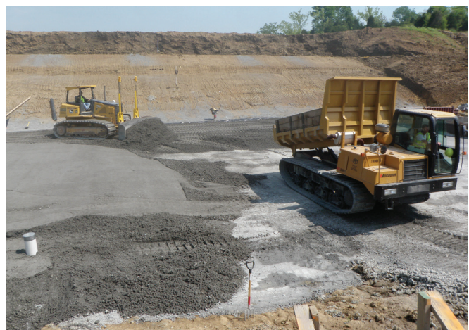
FIGURE 9-6. Haul truck delivering fresh RCC to the placement area.
