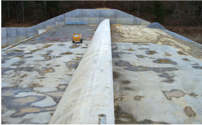
FIGURE 6-22. Ogee crest weir (Fox Creek MPS No. 4, KY).
