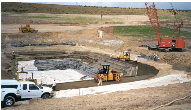
FIGURE 9-11. RCC placement using concrete bucket lifted by crane.
