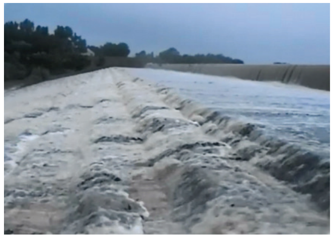
FIGURE 10-6. Overtopping spillway activated during storm event (Leyden Dam, CO).
