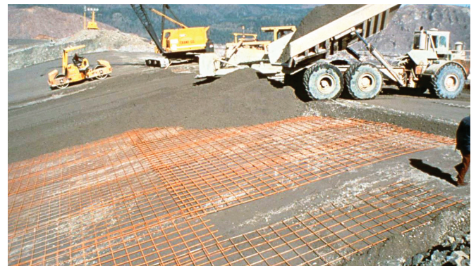
FIGURE 6-5. RCC plated spillway (Toutle River Dam, OR).
