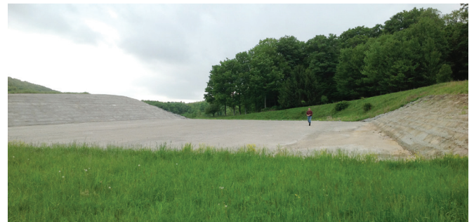
FIGURE 6-6. RCC plated armoring of auxiliary spillway (North Fork Dam, PA).
