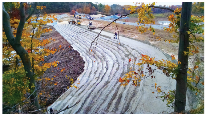
FIGURE 6-9. Unformed RCC chute with compacted RCC (Speedwell Forge Lake Dam, PA).
