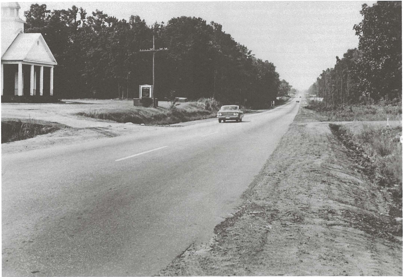
Constructed in 1935, the first scientifically controlled soil-cement project, SC 41 near Johnsonville, South Carolina, after 30 years of service (1965 photo).
