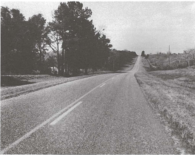
A soil-cement road in Florida
