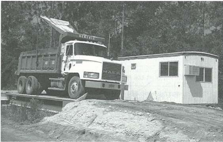
Fig. 14. Each load of soil-cement from a central mixing plant is weighed for a continuous record of the quantity processed. Note tarp being placed over the soil-cement to minimize evaporative moisture lost during transport. Covering soil-cement also protects it from rain.
