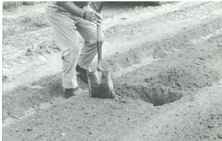
Fig. 22. Uniform color indicates thorough mixing.
