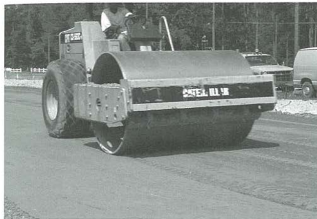
Fig. 24. Compacting the soil-cement with a vibratory steel wheel roller.
