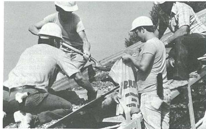
Fig. 12. Collecting soil material from main feeder belt to determine dry weight and rate of feed.
