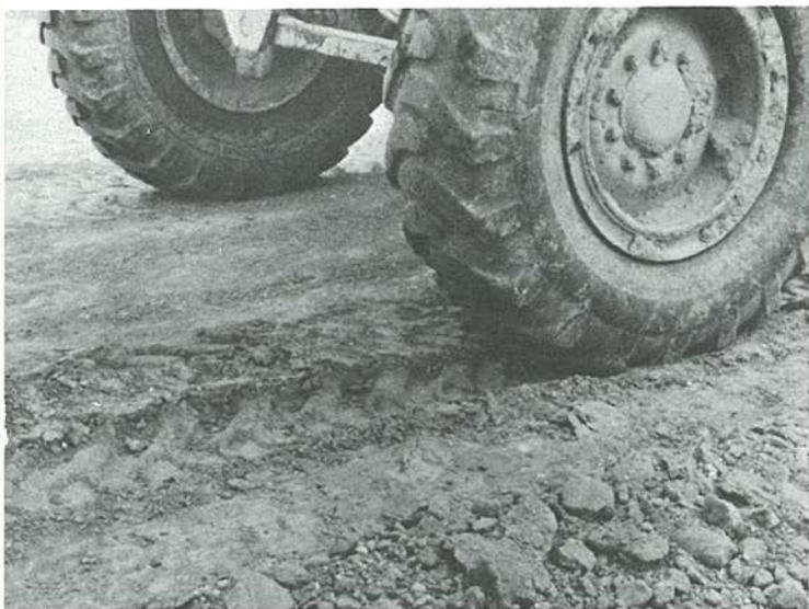
Fig. 2. Unstable subgrade areas can usually be detected by observing their stability under the motor-grader wheels. Soft areas must be corrected before processing starts.
