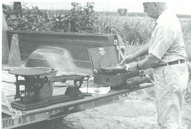
Fig. 19. Soils are dried on a portable stove to determine moisture content.
