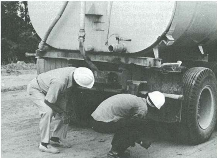
Fig. 3. Checking for water truck spraybar leakage.
