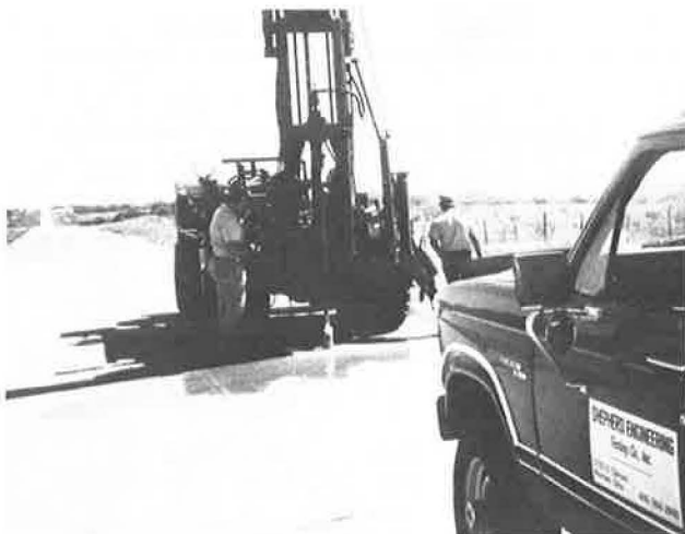
FIGURE 1 CME 750 coring the concrete pavement.
