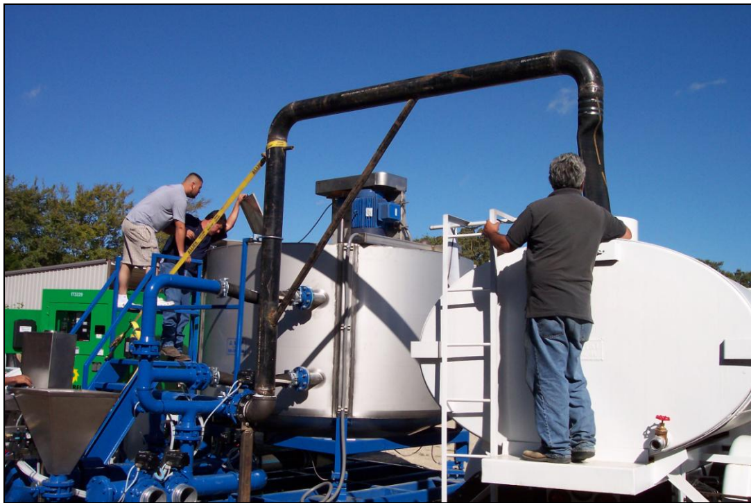
Figure 1.10. Texas Slurry Batch Plant Offloading Slurry into Spreader Truck.
