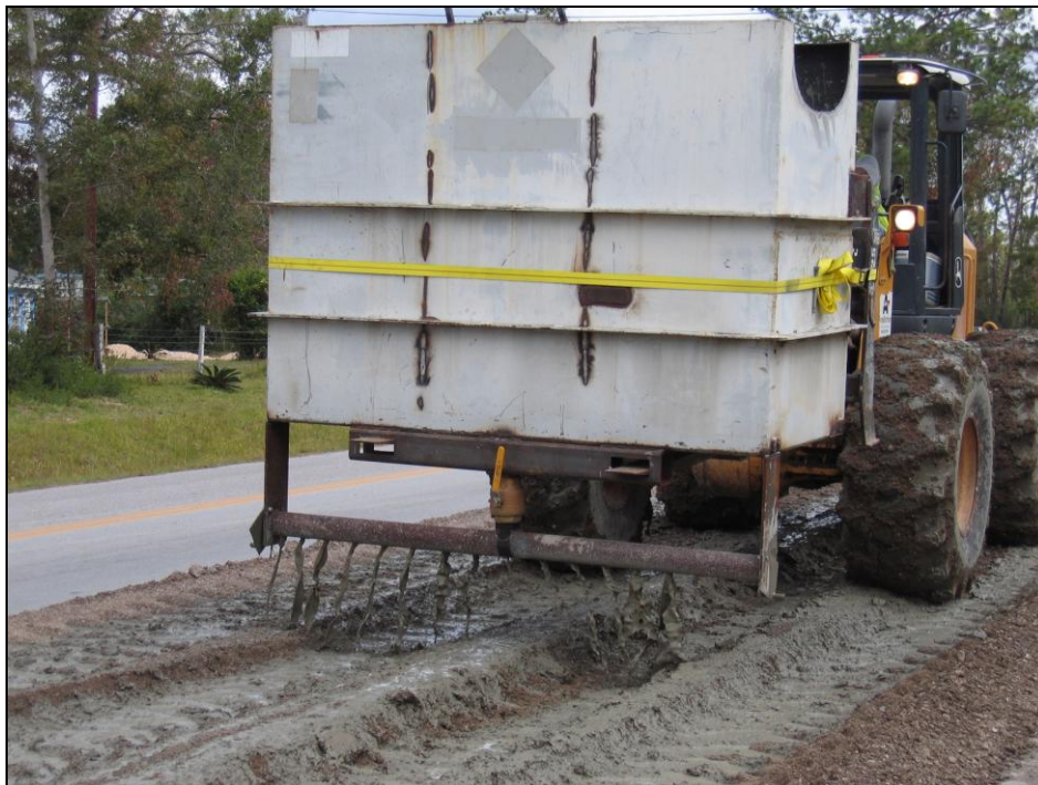
Figure 1.7. Spreading Slurry with the Angel Brothers Spreader Box.
