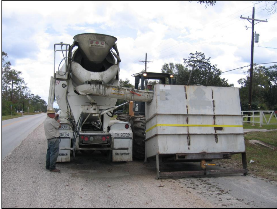
Figure 1.6. Loading Slurry from Cement Truck into Spreader Box.
