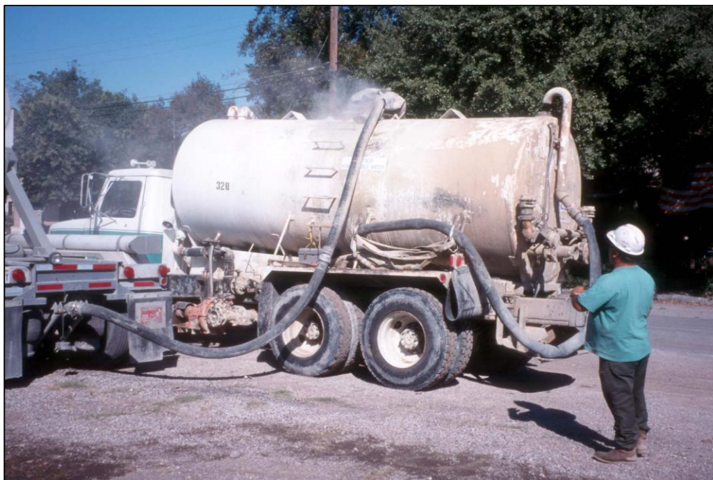
Figure 1.4. Filling the Olmos Construction Slurry Truck with Dry Cement. Note: photo courtesy of Olmos Construction.
