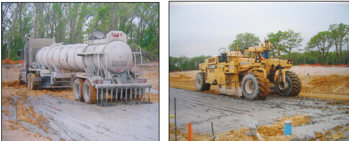
Figure 1.3. Placement and Mixing Super Slurry.
