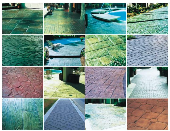
Figure 37. Patterned, textured, and colored concrete can be used anywhere than an attractive durable finish is needed. Several types and applications of pattern stamped finishes are shown. (IMG: 7080, 7081, 7082, 7083, 7084, 7085, 7086, 7087, NA, 7089, 7090, NA, 9001, 9002, 9003, 9004)
