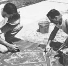
*Figure 47. Removing strips after concrete has hardened. (22758-I)*
