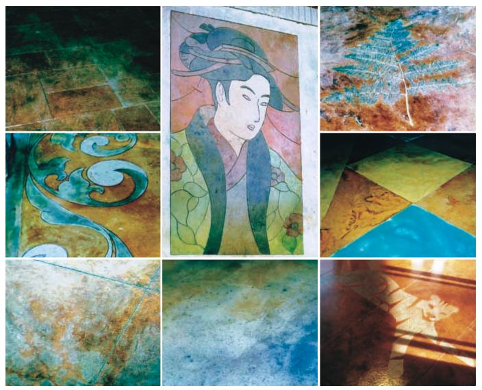
Figure 80 (continued). Examples of colored surfaces using chemical stains, dyes, and tints in combination with a variety of other decorative concrete strategies.
