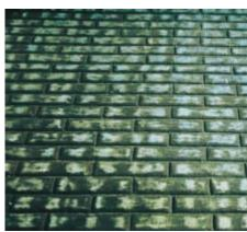
Figure 41. Mottled brick pattern rolled surface produced by grinding off some of the surface. (IMG9020)
