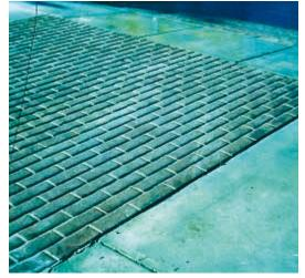
Figure 39. Brick design produced by pattern rolling.
