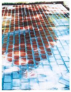
Figure 63. Completed inlaid brick finish after the template has been removed and the surface cleaned of loose particles. (13978)
