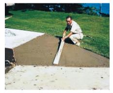
Figure 5. After strikeoff, the surface is leveled and smoothed with a wood darby. A bullfloat also may be used. (13923)
