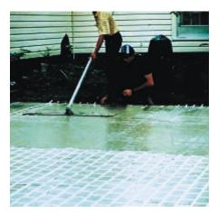
Figure 58. The paper template is embedded with a bullfoat. (13966)
