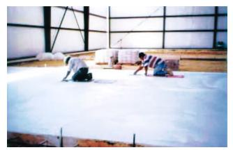
Figure 76. Clean tools are essential for creating light reflective concrete floor surfaces. Hand finishing is recommended for the final pass, as machine finishing can create a burnished appearance, which may not be acceptable. (70104)
