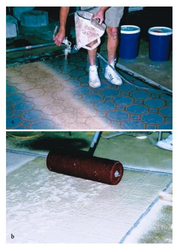
Figure 79. (a) Overlay material is sprayed over a paper stencil to create a relief pattern. (b) A texture roller applied to the surface of a stenciled bonded overlay.
