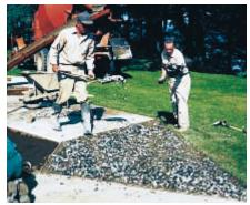
Figure 7. The entire surface must be completely covered with just one layer of the select stone. (13925)
