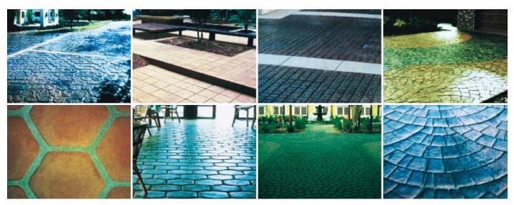
Figure 37 (continued). Patterned, textured, and colored concrete can be used anywhere than an attractive durable finish is needed. Several types and applications of pattern stamped finishes are shown. (IMG: 9005, 9006, NA, 9008, 9009, 9010, 9011, 9012)
