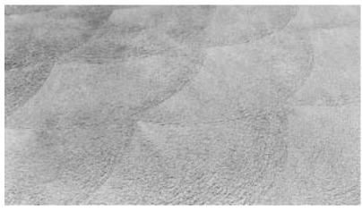
Figure 21. Swirl finish produced with a hand float. (29269)
