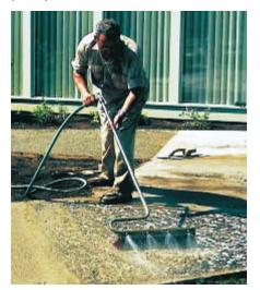
Figure 12. Next, fine spray the surface with water along with brushing. Special exposedaggregate brooms with built-in water jets (pictured) are available. (13930)
