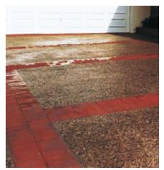
Figure 70. Masonry units of concrete, brick, or rock, used as divider strips and borders may be set in a sand bed with or without mortar joints. (13920)
