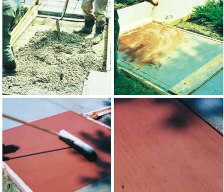
Figure 77. Dry-shake coloring. (a) Concrete is placed, screeded, and floated using conventional techniques. (b) Dry-shake coloring compound is broadcast onto the surface. (c) The dry shake is floated and troweled into the surface. (d) Brooming the surface. (e) Completed dry-shake surface. Also see Figures 52, 59, 60, and 61. (l to r, 13913, 13914, 13902, 13904, 13917)
