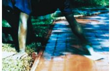
Figure 61. For smooth textures, the surface is then troweled. Broomed, floated, and other textures can also be used. (13969)
