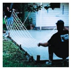
Figure 56. To produce an inlaid brick pattern, a paper template is first trimmed to the width of the slab. (13964)
