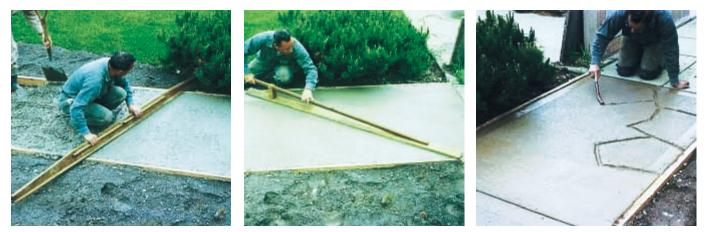
Figure 49. Tooled or incised flagstone. (a) Striking off the concrete. (b) Darbying the surface. (c) Tooling joints into slab to form a flagstone pattern. (IMG9054, 13901, 13909)
