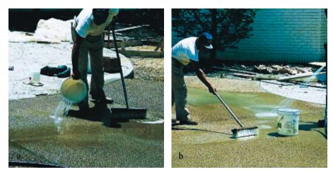
Figure 16. Acid washing to clean the surface. (a) First, a small quantity of muriatic acid (dilute hydrochloric acid) is applied to the hardened, two week old exposed-aggregate surface, which should be in a moist state. (b) The acid solution and brushing will clean the surface of any cement film remaining from the aggregate exposure operation. The acid is then washed away from the surface with water. (13960, 13961)
