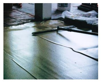
Figure 78. Thin specialty material is applied to accommodate a stamped overlay.
