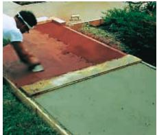
hazardous when wet; therefore, hard steel-troweled surfaces are not recommended for exterior slabs.
