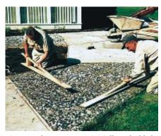
Figure 8. The aggregate is initially embedded by tapping or tamping with a wood darby. A hand float or a straightedge may also be used. (13926)
