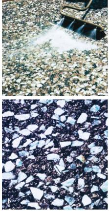
Figure 13. (a) Continue washing and brushing until flush water runs clear and there is no noticeable cement film left on the aggregate. (b) Close-up view of the completed exposedaggregate surface. (13931, 13932)
