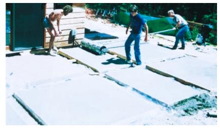
Figure 38. Pattern rolling uses a cylinder with a pattern relief on it to impress a design into the concrete surface. (13977)
