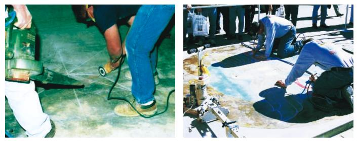
Figure 73. (a) Scoring patterns with a hand held grinder equipped with a diamond blade. (b) Mechanically controlled concrete router for intricate design work.
