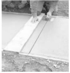
Figure 71. When scoring or jointing with a groover, the use of a straightedge such as a board 25-mm (1-in.) thick and at least 150-mm (6-in.) wide is recommended as a guide. (23227-B)
