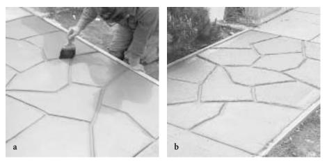
Figure 50. Troweling after jointing and floating. A floated surface is usually satisfactory for exterior applications. (22758)
