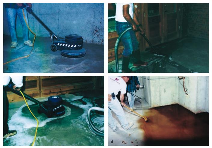
Figure 81. (a) Sanding a concrete surface in preparation to receive stains, dyes, or tints. (b) Washing the surface prior to stain, dye, or tint application. (c) Vacuuming wash water to assure a clean surface. (d) A typical application method when a single color stain is used.
