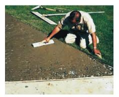
Figure 10. Final embedment is done with a hand float until appearance of the surface is similar to that of a normal slab after floating. (13928)
