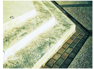
Figure 31. (a) Silicon carbide grains are lightly troweled into the surface of a municipal sidewalk. (b) Nonslip aggregate on steps. (P-23352-B, IMG7078)
