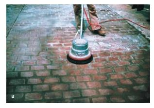
Figure 36. (a) After the grout in the joints has set, a rotary floor polisher is used to remove the grout residue from the surface. (b) Pictured is grouted fish scale cobblestone pattern used for both interior flooring and exterior paving. (13954, IMG7079)
