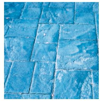
Figure 2. Pattern-stamped finish. (IMG7054)
