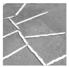
Figure 44. Laying out random flagstone pattern with wooden strips. (22758-K)
