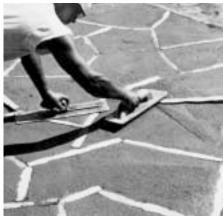
Figure 45. Floating in wooden strips.
