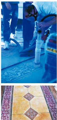
Figure 66. (a) Stencil and sandblasting operation. (b) Finished sandblast stencil example.
