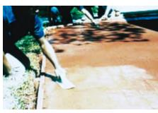
Figure 60. The color is worked into the surface with a hand float, as shown, or a bullfloat, depending on the size of the slab. (13968)
