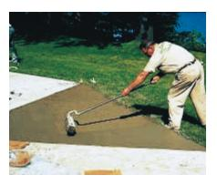
Figure 11. In exposing the aggregate, timing is critical. Work should begin as soon as the mortar can be removed without over-exposing or dislodging the aggregate. The first step is to brush the surface lightly with a stiff, nylon bristle broom to remove excess mortar. (13929)
