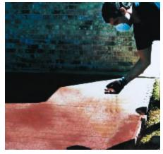
Figure 59. Dry-shake coloring compound is broadcast onto the surface. (13967)
