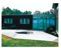
Figure 14. This attractive patio combines contrasting areas of plain broom-textured concrete with panels of black and white exposed aggregate. (13933)
