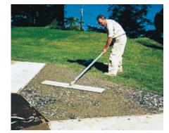
Figure 9. Further embedment of the aggregate is done with a bullfloat. (13927)
