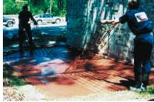
Figure 62. The paper template is removed when the concrete has set sufficiently. (13970)
