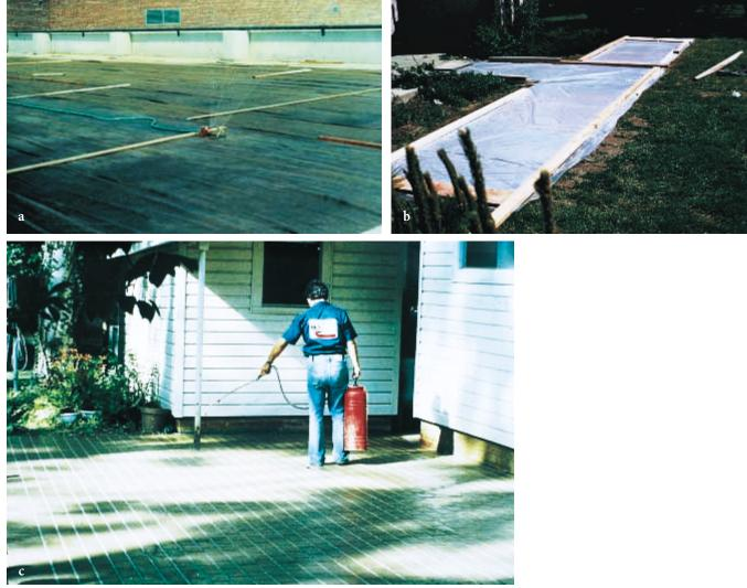
Figure 84. Concrete must be cured to achieve the desired strength and durability. (a) Burlap covering kept continuously moist with a sprinkler. (b) Plastic sheeting prevents moisture from leaving the slab. Plastic sheeting can also be used over wet burlap to keep the burlap moist. (c) A curing compound retards the evaporation of water from the concrete. (12263, 13907, 13973)
