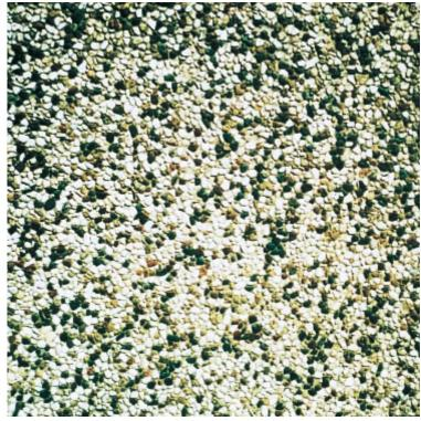
Figure 1. Exposed-aggregate finish. (IMG7053)
