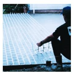
Figure 57. Each piece of template is positioned onto the bullfloated slab adjacent to the previous piece until the entire slab is covered with the template. (13965)
