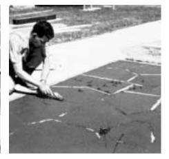
Figure 46. Cleaning wooden strips. (22758-G)
