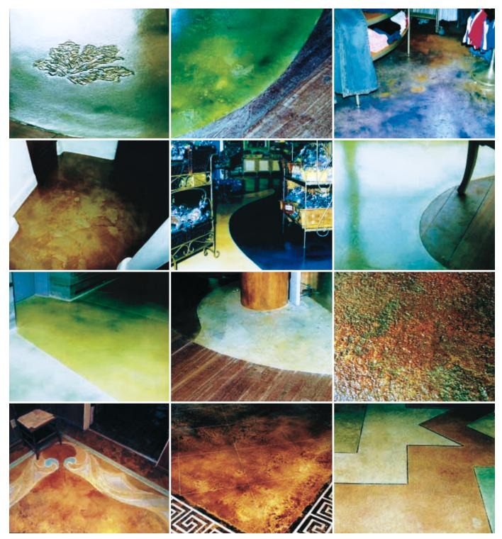
Figure 80. Examples of colored surfaces using chemical stains, dyes, and tints in combination with a variety of other decorative concrete strategies.
