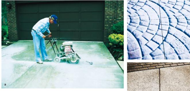
Figure 82. (a) Saw cutting a contraction joint in a driveway. (b) Saw-cut joint in pattern stamped concrete. (c) Hand-grooved joint in an exposed-aggregate concrete. (a through c: 13971, 13972, IMG9040)
