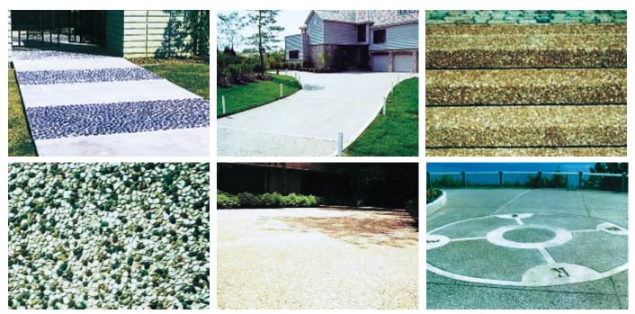
Figure 18 (continued). Various applications and textures obtained with exposed-aggregate concrete. (l to r, IMG7059, IMG7064, 13963, IMG7053, IMG70707, NA)
