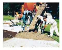
Figure 3. Concrete to receive a seeded exposedaggregate finish should have a slump of between 75 mm and 125 mm (3 in. and 5 in.). (13921)
