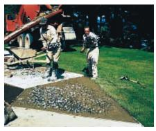
Figure 6. The select aggregate is spread uniformly by shovel and hand. Here a mixture of black and white crushed stone is used. (13924)
