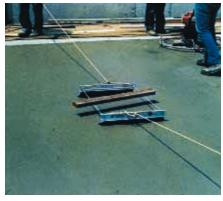
Figure 25. Special double pull broom used to broom long distances. (13943)
