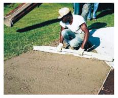
Figure 4. The slab is struck off in the usual manner except that the level of the surface should be left 3 mm to 11 mm ( $\frac{1}{8}$  in. to  $\frac{7}{16}$  in.) lower than the top of forms to accommodate the seeded aggregate (see Table 2). (13922)
