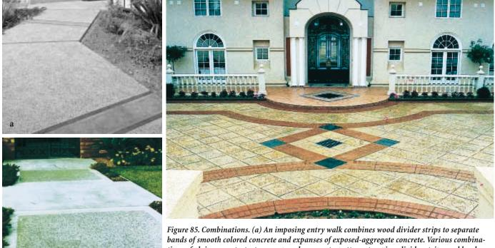
Figure 85. Combinations. (a) An imposing entry walk combines wood divider strips to separate bands of smooth colored concrete and expanses of exposed-aggregate concrete. Various combinations of plain concrete, textures, exposed aggregate, pattern stamping, divider strips, and borders are shown in the other views. (l to r, 21724, IMG: 9046, 9042, next page, l to r, IMG: 9044, 9045, 9043, 9047, 9048)
