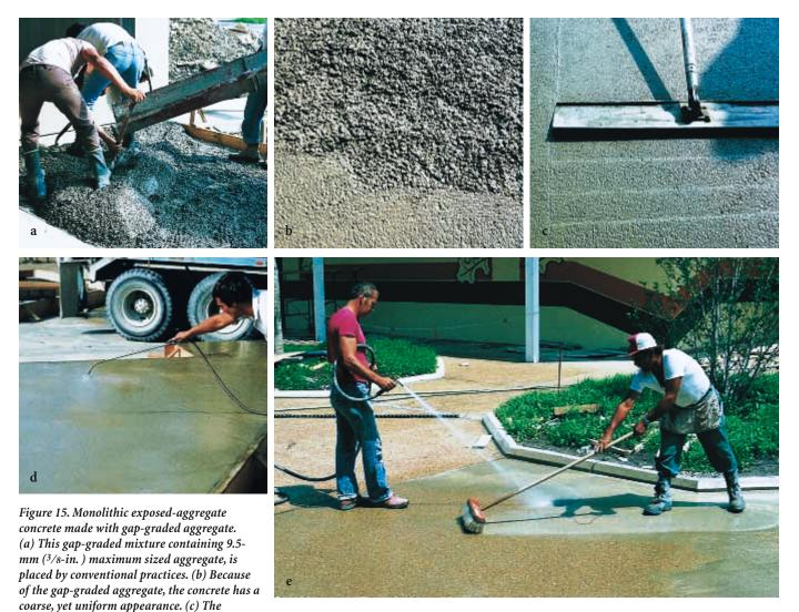
concrete is screeded and then bullfloated and hand floated. (d) A surface retarder is sprayed on the surface to ease mortar removal. (e) After the concrete is hard enough to walk on and retain the coarse aggregate, the surface is washed and brushed to expose the aggregate. (13956, 13957, 13958, 13959, 10098)
