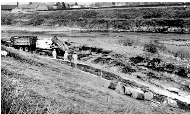
Fig. 2. Cement-bentonite slurry trench being installed for Superfund project in Pennsylvania.
