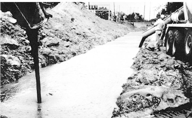
Fig. 4. Backfilling utility cut trench with Controlled Low Strength Material (CLSM).
