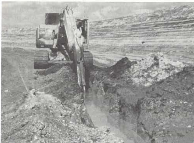
Fig. 36. Cement-bentonite slurry-trench construction. Reference 38.
