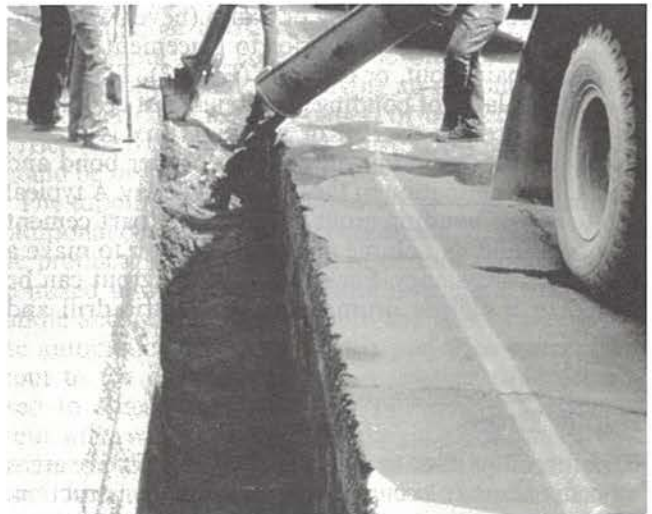
Fig. 24. Flowable fill used to backfill a utility trench along a street.
