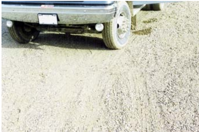
Figure 8. Free-draining, unstabilized subbase with enough fines to be stable during construction but still provide permeability of about 200 ft/day (60 m/day) in laboratory tests. Note that the truck tires are not causing excessive rutting or displacement of the subbase material.
