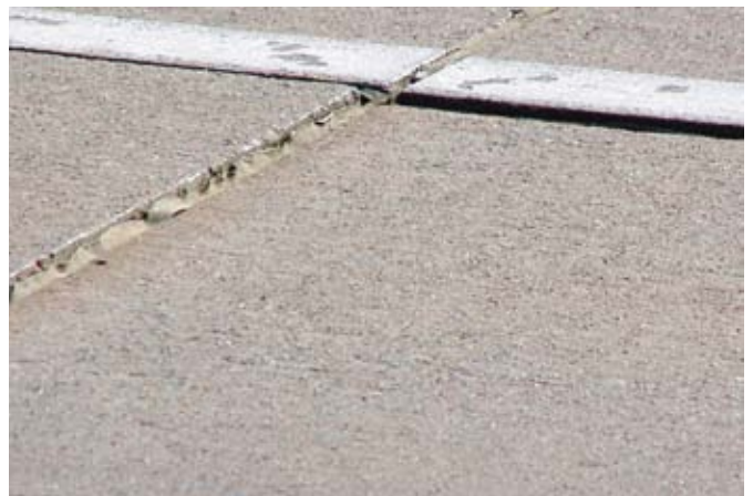
Figure 32. Faulted joint.
