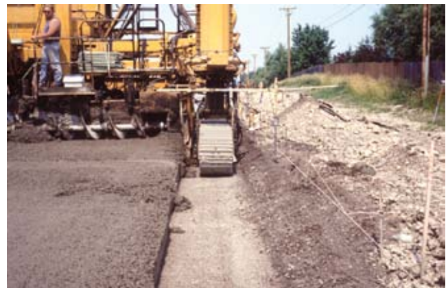
Figure 33. Trackline for slipform paving machine.
