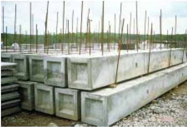
Figure 3.23. Precast concrete blocks used to construct face of spillway at Big Haynes Dam, GA.
