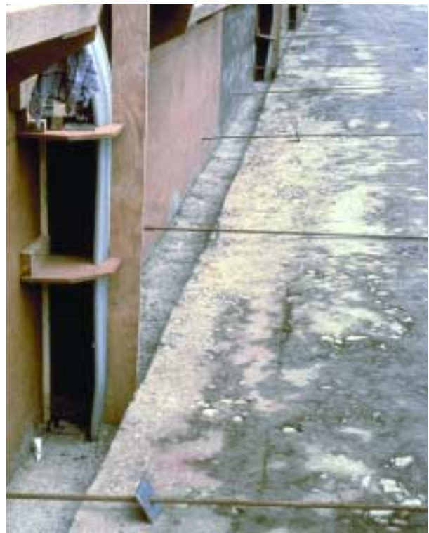
Figure 2.9. Installation of waterstop at vertical joints, Monksville Dam, NJ.
