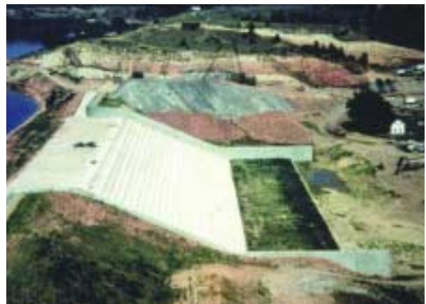
Figure 3.19. Completed RCC stepped spillway at Tongue River Dam, MT.
