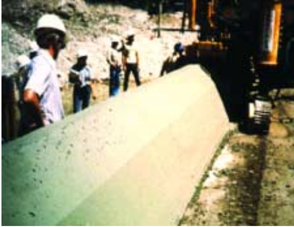
Figure 2.23. Casting of slip-formed facing element.
