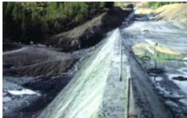
Figure 3.27. Slip-formed downstream face, Elk Creek Dam, OR.
