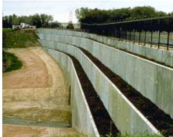
Figure 3.21. Downstream face of North Loop Detention Dam, TX.
