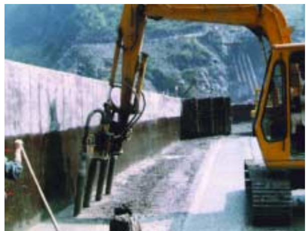
Figure 2.36. Placement and internal vibration of grout-enriched RCC at Jiangya Dam in China (photo courtesy of William A. Moler).
