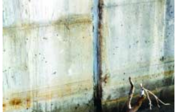
Figure 2.8. Vertical notch with sealant, New Elmer Thomas Dam, OK.
