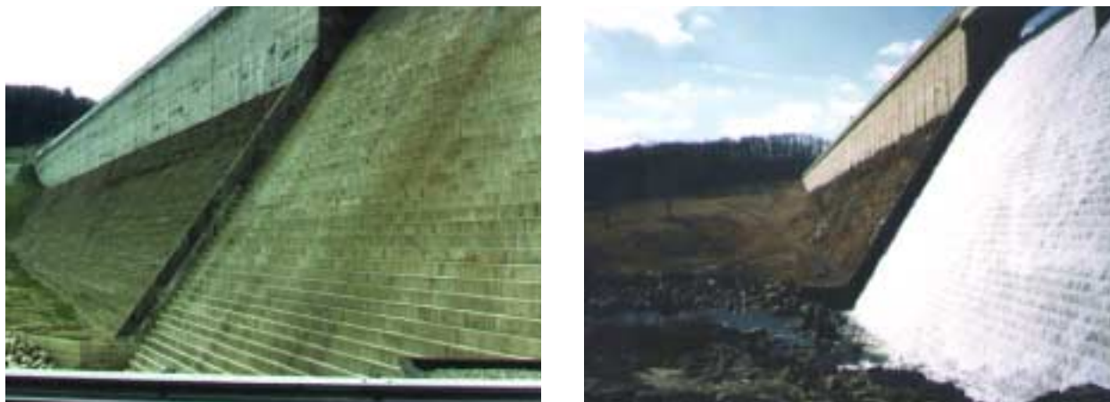
Figure 3.2. Formed conventional unreinforced concrete spillway steps, Monksville Dam, NJ.
