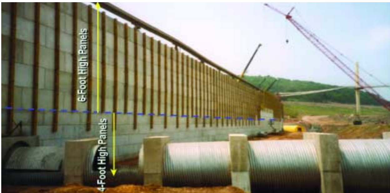
Figure 2.21. Construction photo of upstream face of Penn Forest Dam, PA.
