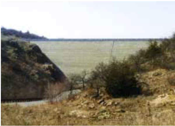
Figure 3.13. Formed conventional concrete face, New Elmer Thomas Dam, OK.
