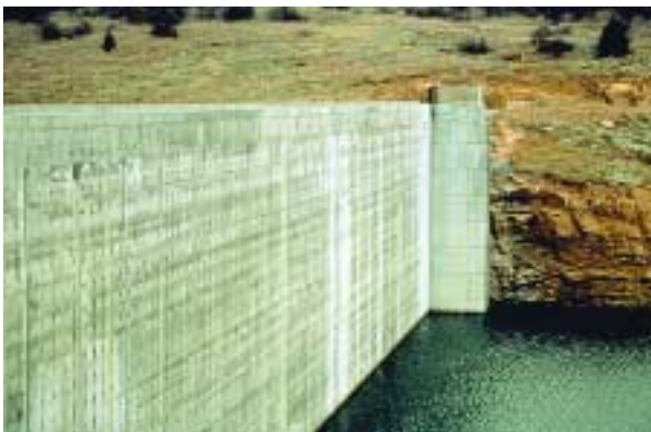
Figure 2.7. Upstream face of New Elmer Thomas Dam, OK.
