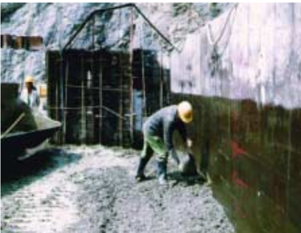
Figure 2.36. Placement and internal vibration of grout-enriched RCC at Jiangya Dam in China (photo courtesy of William A. Moler).
