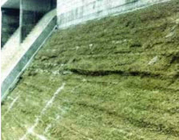
Figure 3.5. Unformed RCC face, Monksville Dam, NJ.
