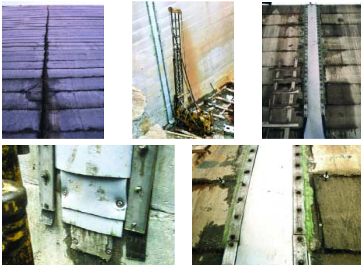
Figure 2.34. CARPI external waterstop system (photographs courtesy of CARPI).
