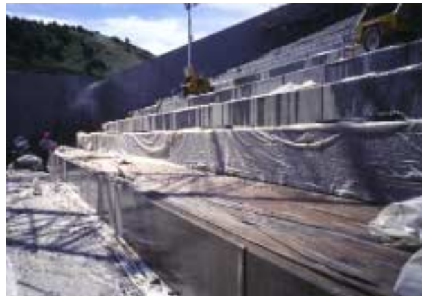
Figure 3.18. Precast panels used to construct steps at Tongue River Dam, MT.
