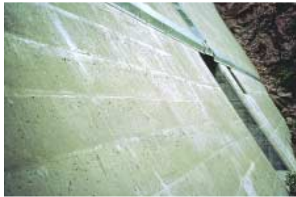
Figure 3.15. Formed conventional concrete face of New Elmer Thomas Dam, OK.
