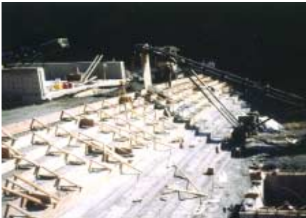
Figure 3.9. Formed RCC face, Long Run Dam, PA.
