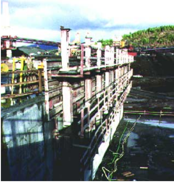
Figure 2.5. Elk Creek Dam, OR.
