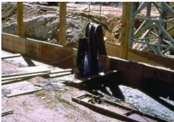
Figure 2.11. Waterstopped contraction joint at Quail Creek Dam, UT.
