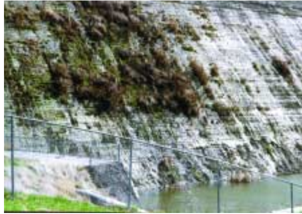
Figure 3.7. Unformed RCC face with vegetation, Willow Creek Dam, OR.
