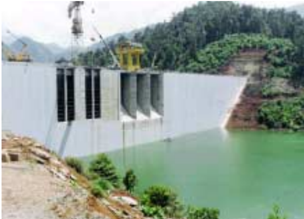
Figure 2.32. CARPI liner system on Balambano Dam, Indonesia.
