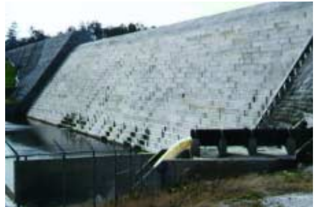
Figure 3.24. Precast concrete block spillway face, Big Haynes Dam, GA.
