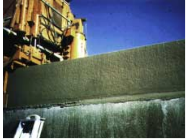
Figure 2.22. Slip-formed facing, Upper Stillwater Dam, UT.
