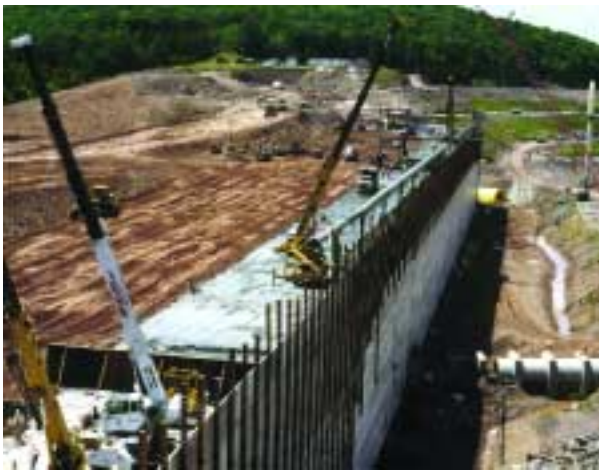
Figure 3.29. RCC placed concurrently with earth fill, Penn Forest Dam, PA.
