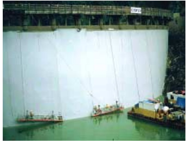
Figure 2.28. CARPI PVC liner system being installed on Lost Creek Dam, CA.
