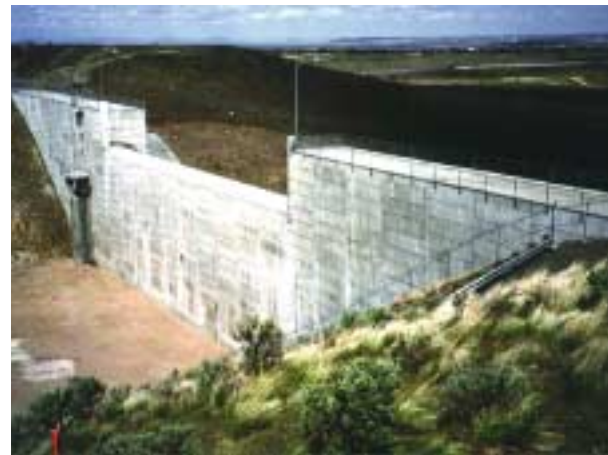
Figure 2.14. Upstream face of Zintel Canyon Dam, WA.
