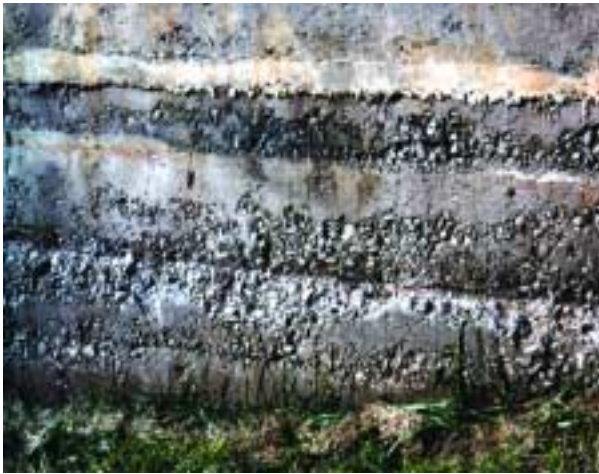
Figure 2.3 Formed RCC (below average quality).
