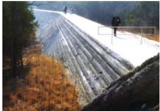
Figure 3.11. RCC slip-formed face, Woody Branch Dam, TX.
