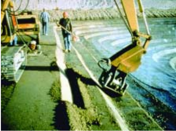
Figure 3.31. Mechanically compacted unformed RCC.
