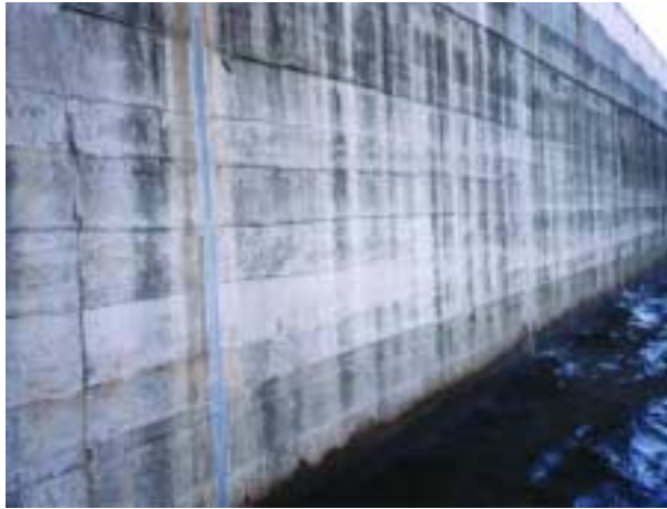
Figure 2.10. Formed unreinforced conventional concrete face of Monksville Dam, NJ.
