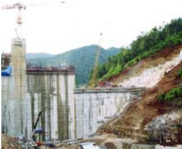
Figure 1.3. Monolithic construction of Balambano Dam, Indonesia.
