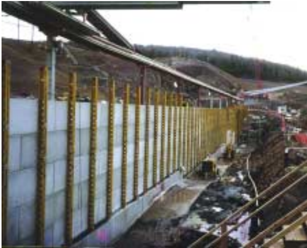
Figure 2.15. Upstream face of Penn Forest Dam, PA showing support of precast panels using strongbacks.
