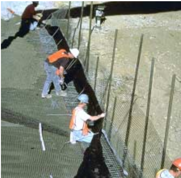
Figure 2.39. Construction of upstream face of Barnard Creek Dam, UT.
