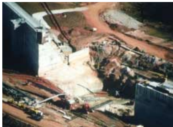
Figure 1.2. Monolithic construction of Big Haynes Dam, GA.
