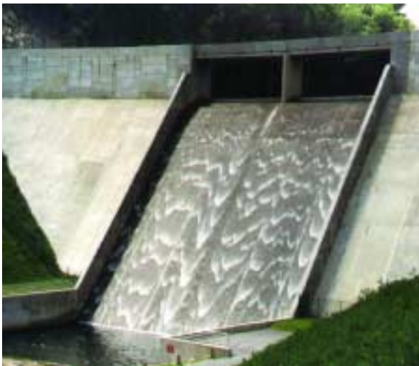
Figure 3.26. Reinforced concrete facing placed after RCC, Siegrist Dam, PA.
