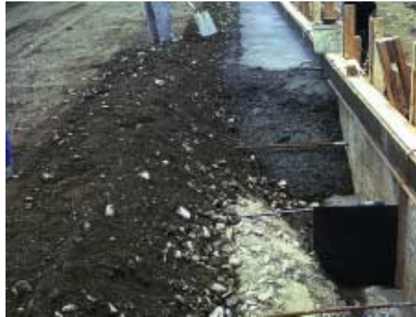
Figure 2.10. Formed unreinforced conventional concrete face of Monksville Dam, NJ.
