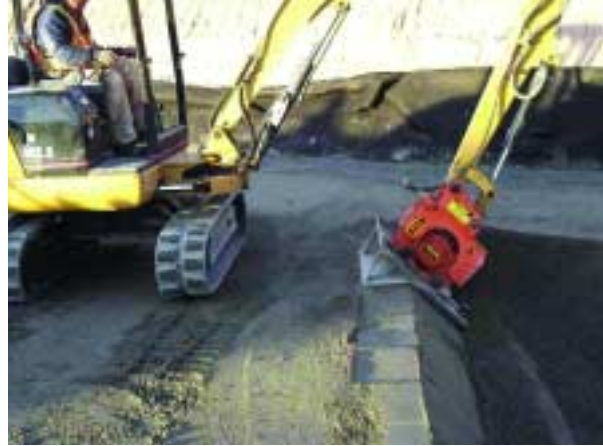
Figure 3.32. Mechanically compacted unformed RCC (photo by Barnard Construction).
