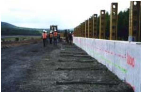
Figure 3.16. RCC against precast concrete panels.
