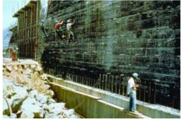
Figure 2.26. Freese Dam, TX.
