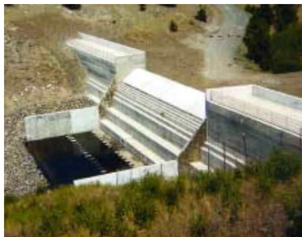
Figure 3.3. Downstream stepped face of Bullard Creek Dam (photo courtesy of Benjamin Doerge).
