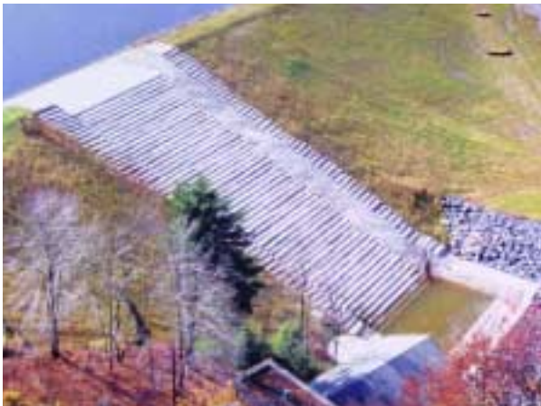
Figure 3.1. Unformed RCC stepped spillway, Ringtown Dam No. 5, PA.
