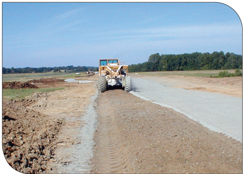
Figure 2 – Mixer incorporating portland cement to a depth of 16 inches
