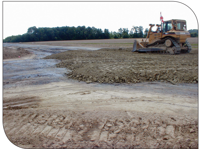
Figure 4 – Embankment being placed easily over cement-modified soil
