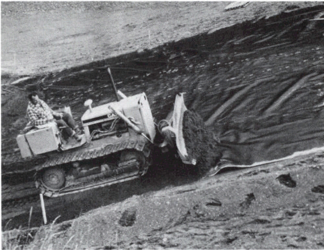
Fig. 9. Spreading soil-cement on membrane at 3:1 slope, Apalachin, N.Y.
