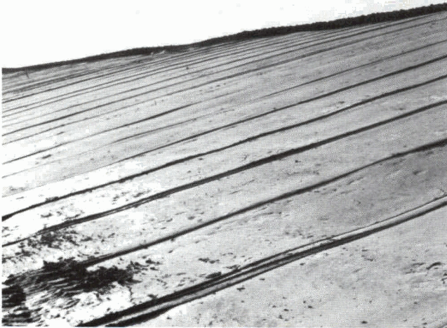
Fig. 2. Completed soil-cement facing at McClellan Site No. 10 Dam, Texas.
