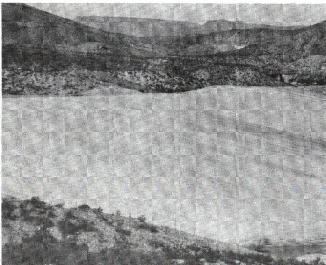
Fig. 3. Soil-cement emergency spillway at Broad Canyon Dam, near Radium Springs, N.M.
