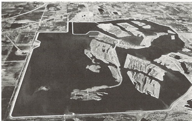
Fig. 3. Aerial view of cooling water reservoir at Braidwood Nuclear Power Station, III.
