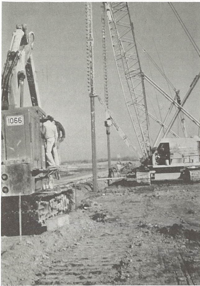
Fig. 10. Two kelly-guided clamshells excavating deep portion of slurry trench. Initial 50-ft depth being excavated with modified backhoe in foreground. Braidwood Power Station, Ill.
