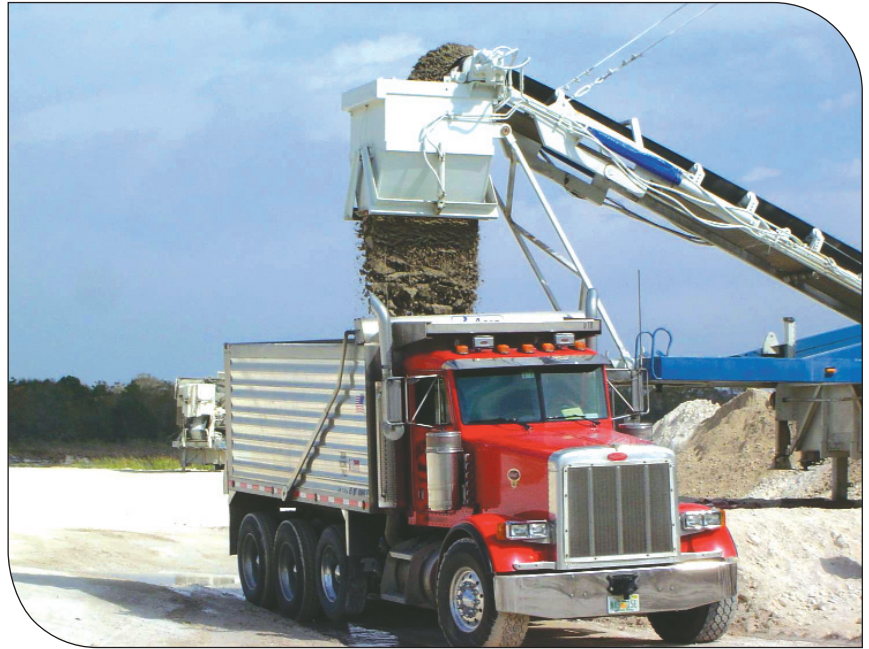
Figure 10—RCC Loaded into Truck for Delivery to Project.
