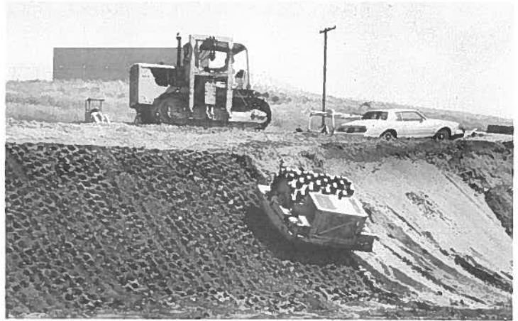
Compacting soil-cement with vibratory sheepfoot roller
