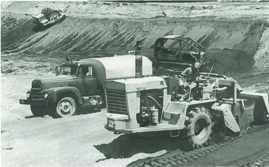
Constructing soil-cement liner.
