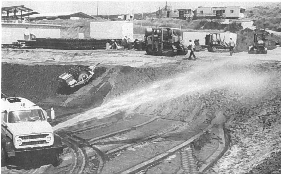
Keeping soil-cement moist prior to compaction.
