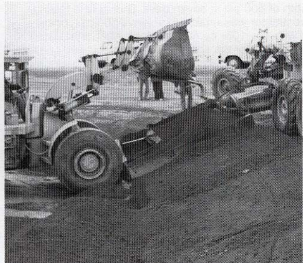
Soil-cement is placed along the slope using special spreader box.
