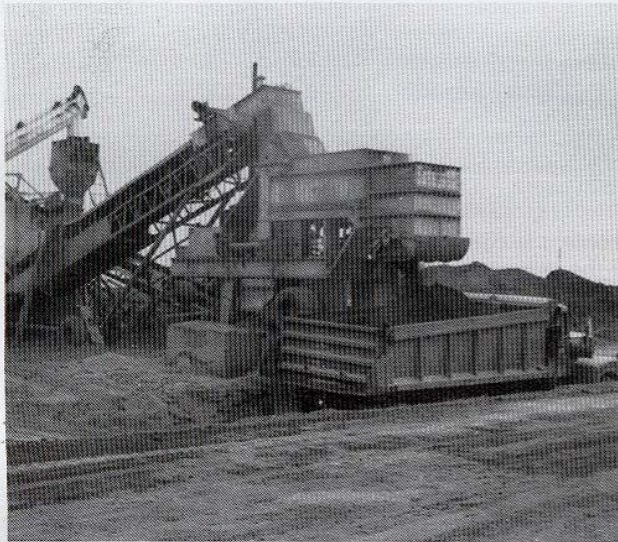
Soil-cement is mixed in continuous-flow central plant.
