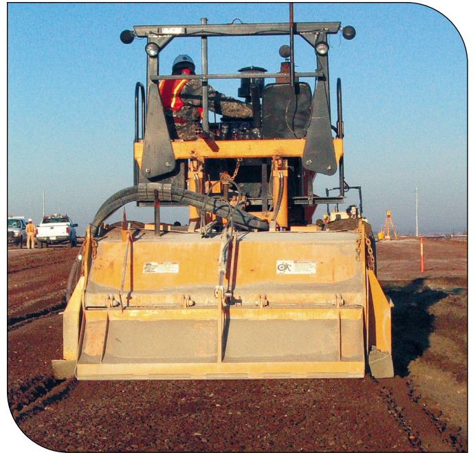
A pulverizer mixes cement into raw subgrade to reduce plasticity levels.
