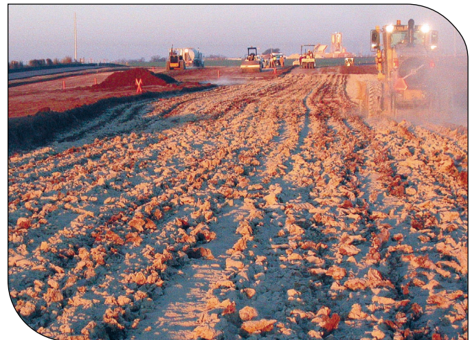
Zachry crews scarify a cement-treated area during subgrade preparation on TxDot's Spur 66 project in San Antonio.
