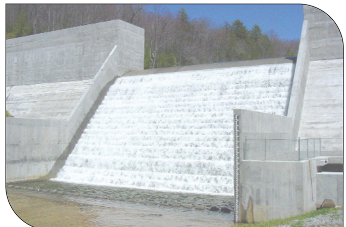
Spillway operating for the first time in April 2006
