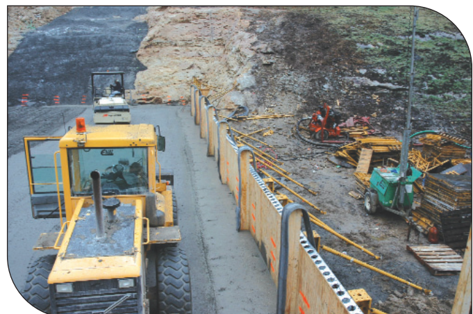
Water stops and conventional concrete facing on upstream face of dam
