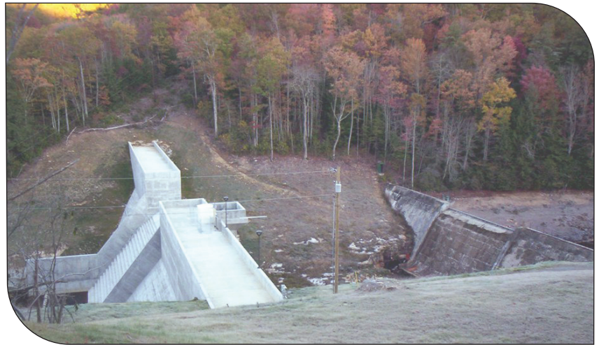
Big Cherry Dams soon after construction of the new dam.
