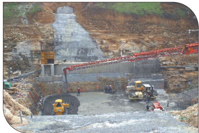
Placement of lower RCC lifts
