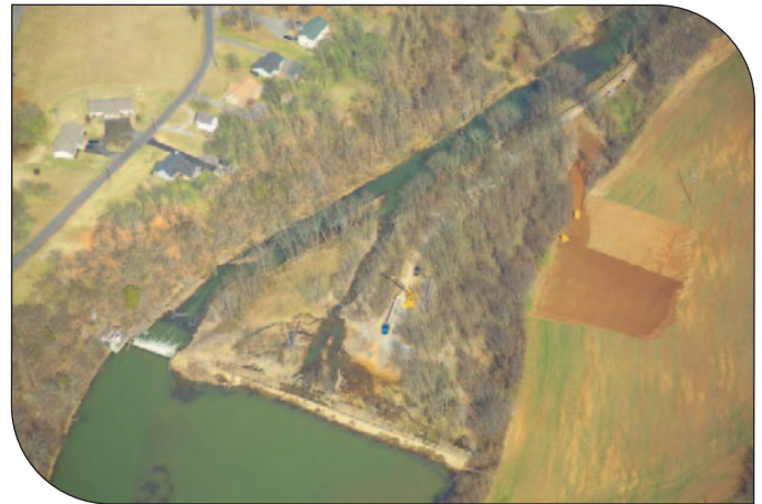
Aerial view of old dam prior to construction
