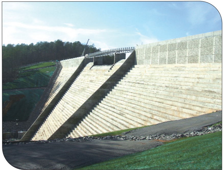
Completed Hickory Log Creek RCC Dam.
