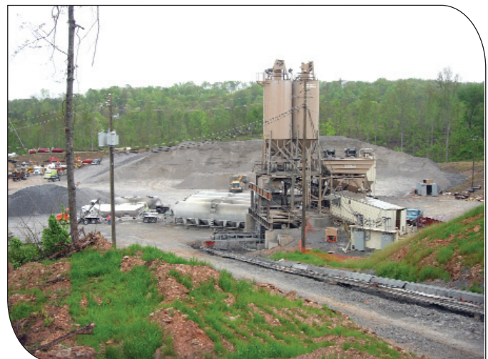
RCC plant and aggregate stockpiles.
