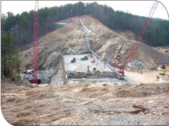
General view of RCC conveying system and placement.
