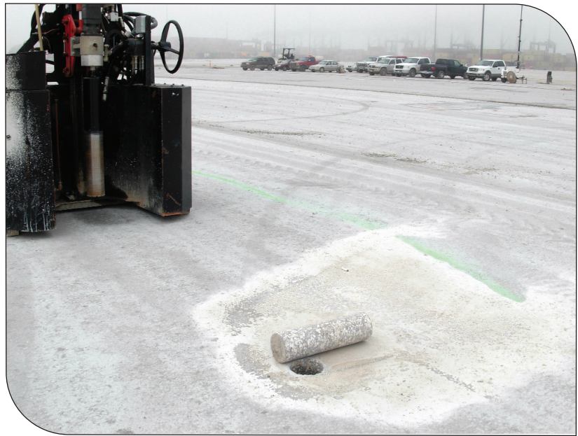
Extracted RCC core for quality control observations and testing
