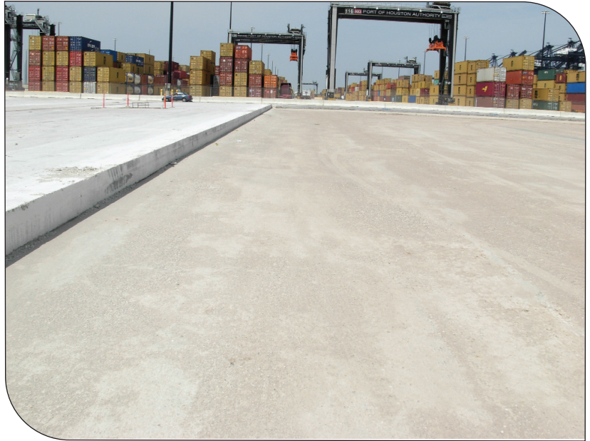
Compacted CTB ready to receive RCC surface
