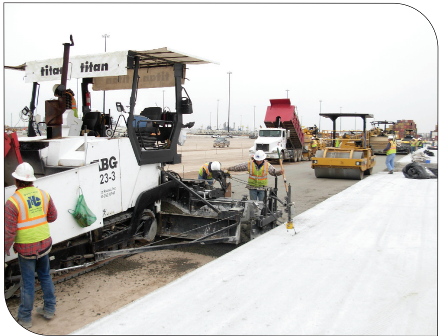
RCC placement at the Port of Houston
