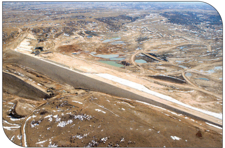
Rueter-Hess Dam under construction in November 2006 . (by Jackie Shumaker Photography)
