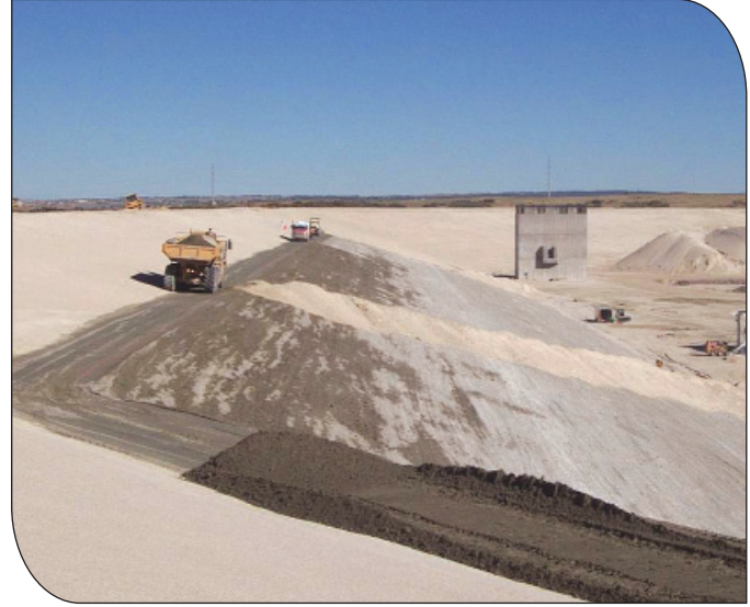
Strair-step construction with unformed step edges . (by Gears, Inc.)
