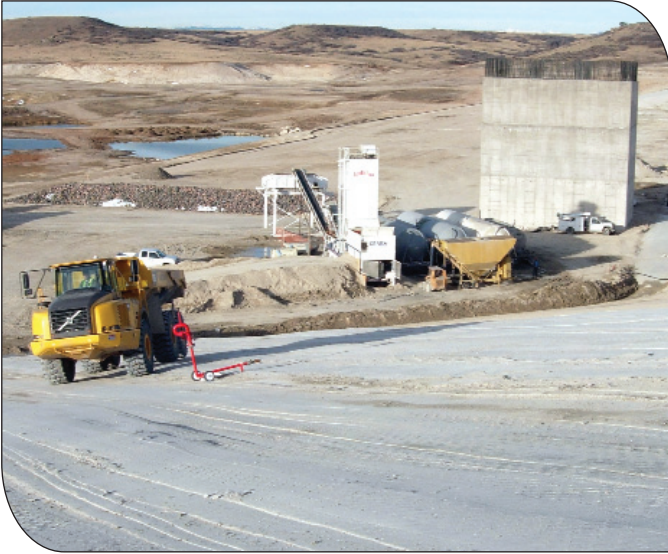
Plated soil-cement and on-site soil-cement mixing plant.
