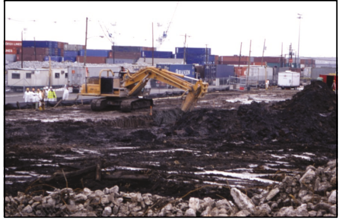
Figure 2. In situ S/S treatment at a former wood preserving facility in Port Newark, NJ.
