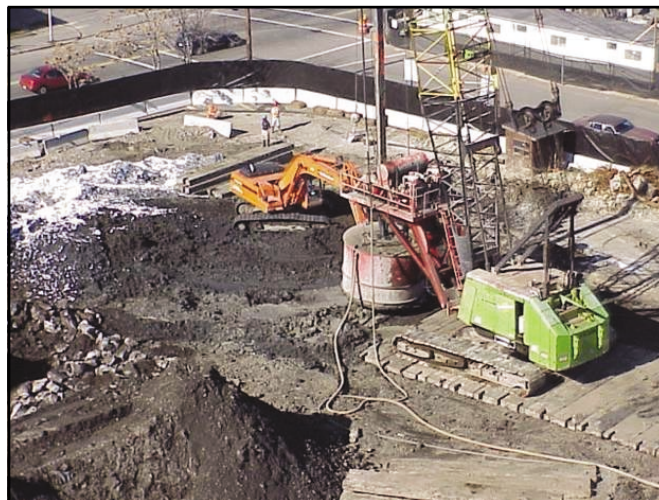
Figure 4. S/S treatment at a former MGP site in Cambridge, MA.
