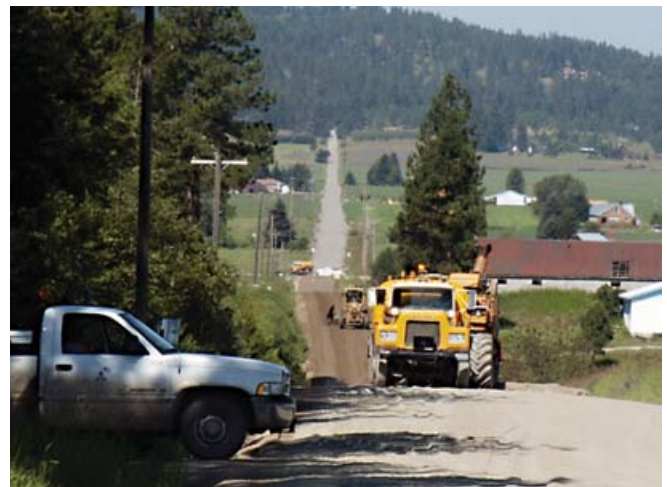
Figure 8. FDR with cement construction, Spokane County, WA.
