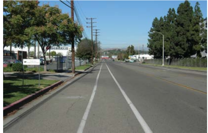
Figure 7. Acacia Avenue Located in an Industrial Zone; Fullerton, California.
