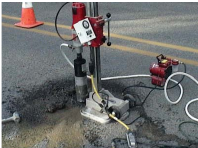
Figure 3. Coring FDR with Cement Roadways.
