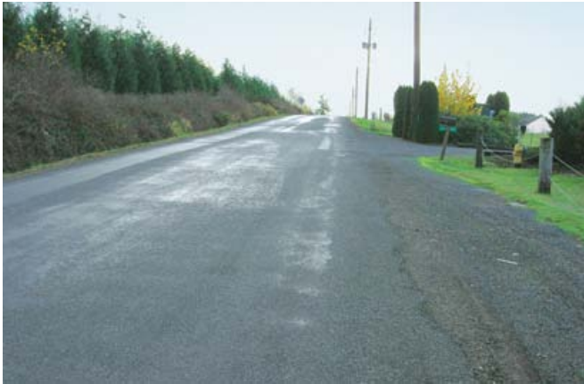
Figure 19. NE 314th Street, Clark County, Washington.
