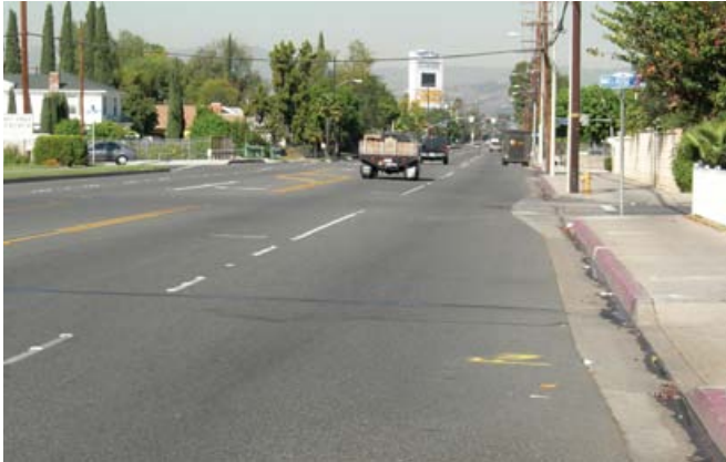
Figure 1. Western Avenue, Buena Park; Orange County, California.
