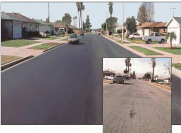
Figure 12. Before and after photos of FDR with cement roadway in Westminster, CA.
