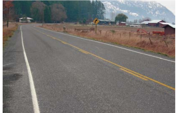
Figure 23. Williams Lake Road, Stevens County, Washington.
