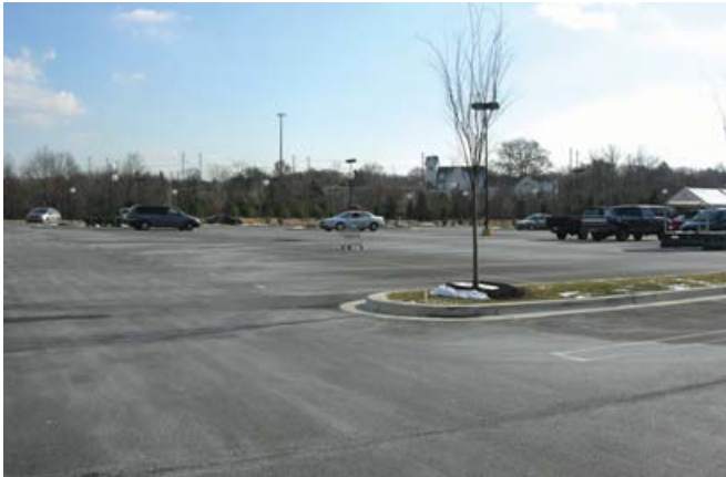
Figure 13. East Gate Shopping Center; Glendale, Maryland.
