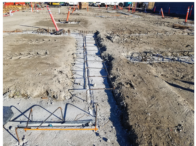
© 2020 Pavement Recycling Systems (PRS) Inc., used with permission
