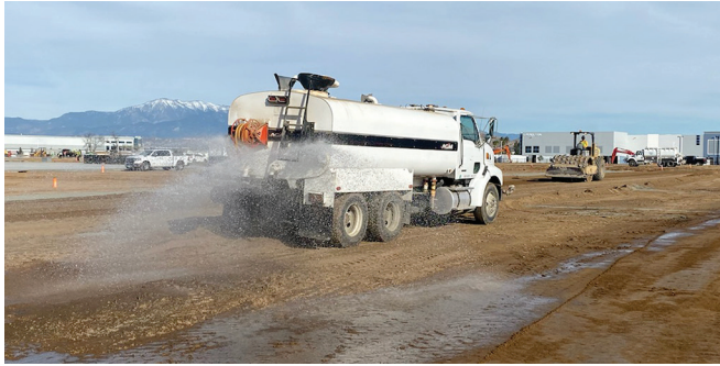
© 2020 Pavement Recycling Systems (PRS) Inc., used with permission
