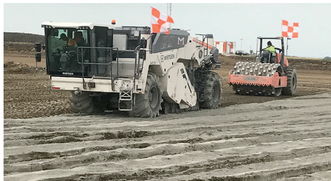
Figure 6.8. Mixing and compacting cement and subgrade
