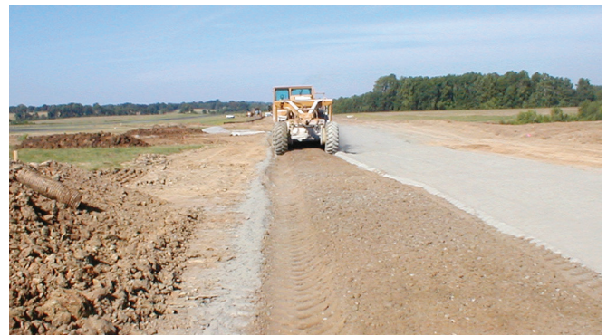
Figure 6.6. Mixer incorporating portland cement to a depth of 16 in.
