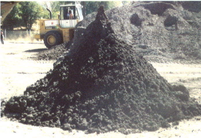
Treated soil as discharged from S/S treatment system.
