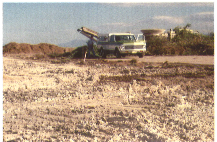
Treated soil (foreground) to be used as a pavement base course.
