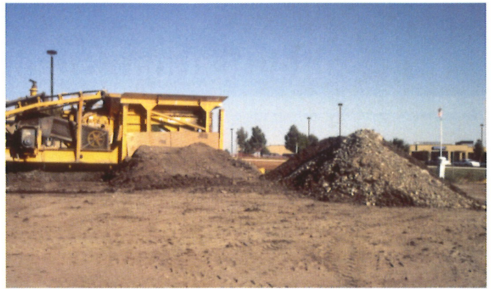
Oversize material awaiting processing by impact crusher.
