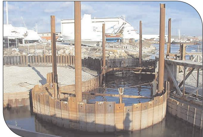
**Steel arcs connecting circular bulkhead cells.**
