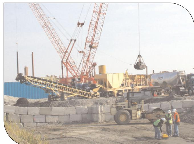
**Dredged sediment placed directly into pugmill mixer.
