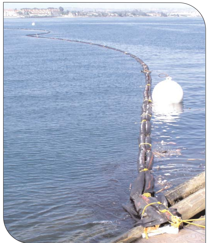
Silt curtain encircles dredge area.
