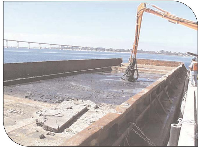
S/S treatment using blending head.
