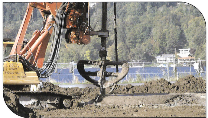
Specially designed auger for soft peaty soils.
