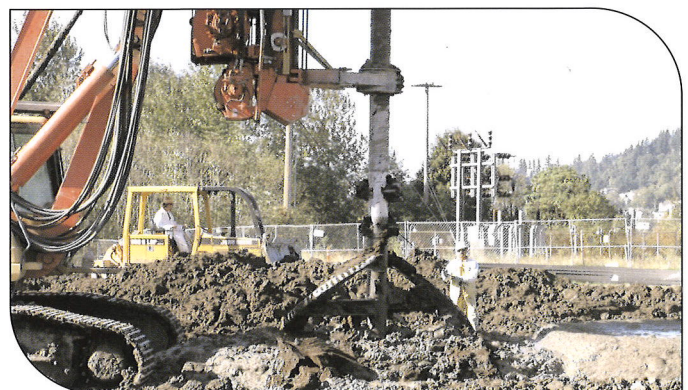
Start of a new mixing column.
