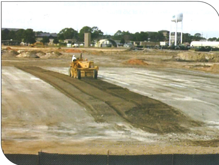
Successive lifts, S/S treated by mixing with road reclaimer
