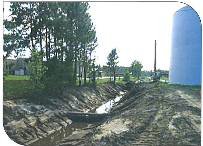
Excavation of sediment from drainage ditches
