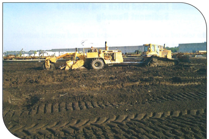
S/S treatment: Mixing by road reclaimer
