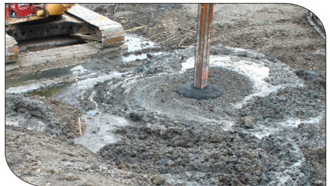
Auger stem markings indicating depth of mixing
