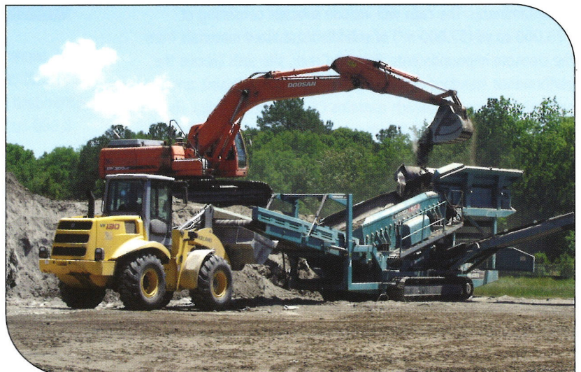
Screening to Remove Oversized Material
