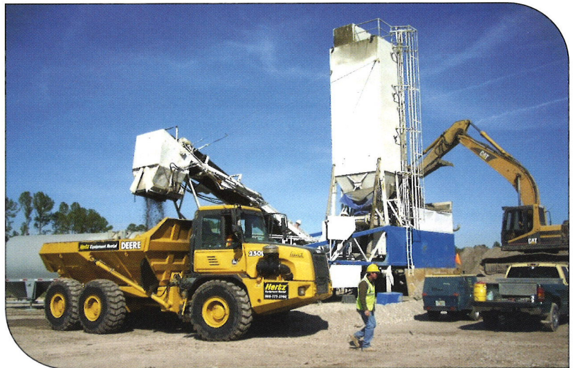
Pugmill Plant On Site
