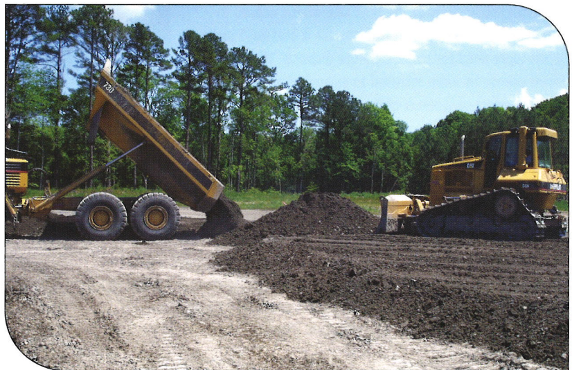
Treated Material Placed as Subcap
