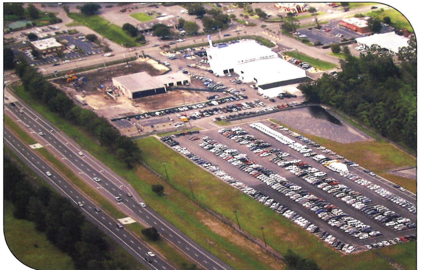
Hercules 009 Landfill after S/S treatment and redevelopment
