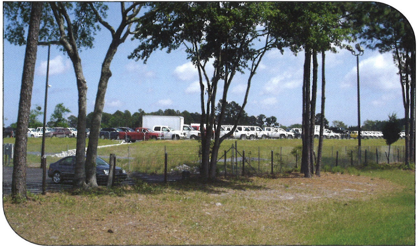
Site capped and paved after S/S treatment (note elevation change)
