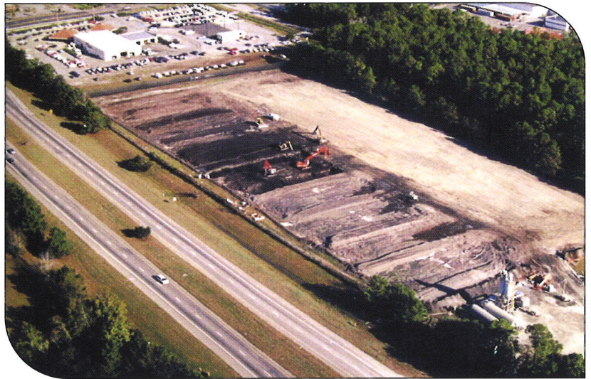
Hercules 009 Landfill during S/S treatment
