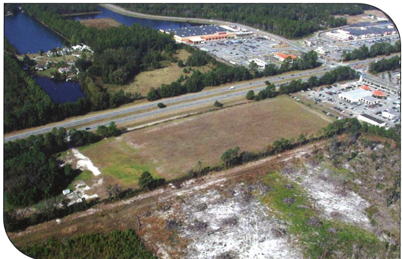
Hercules 009 Landfill after S/S treatment and prior to paving
