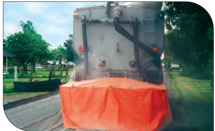
Application of cement.
