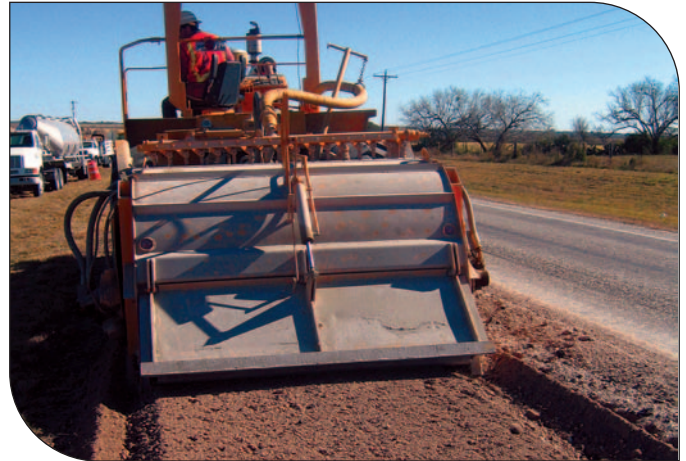
Mixing water and cement into the aggregate-soil mixture.
