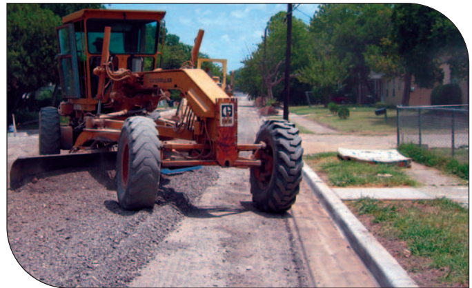
Initial shaping and grading.
