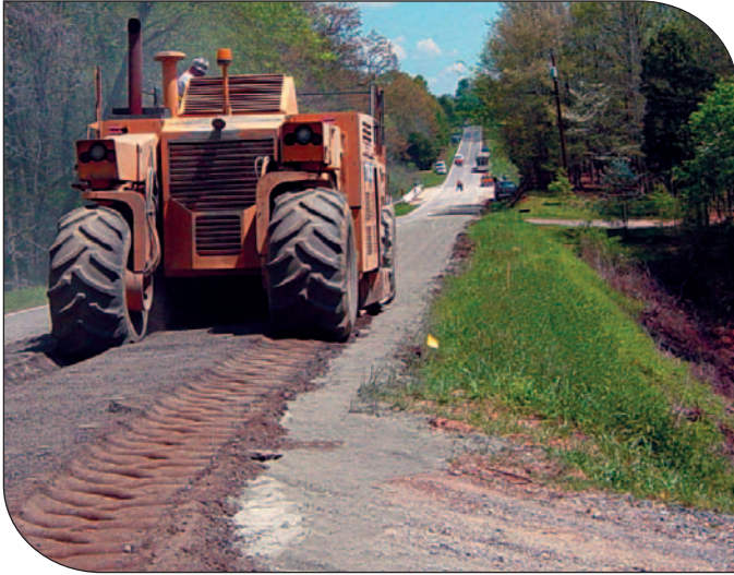
Recycling old asphalt pavement using FDR.
