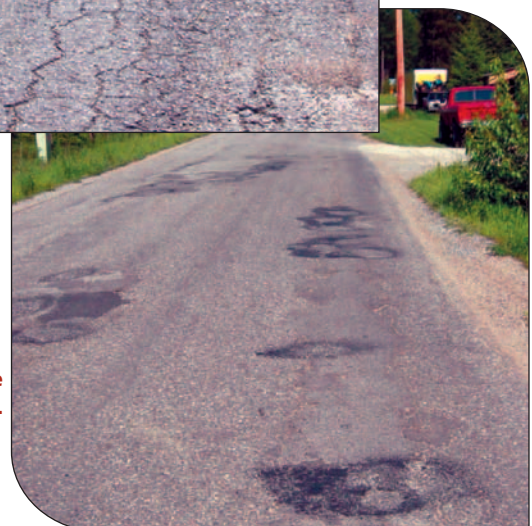
Excessive patching.
