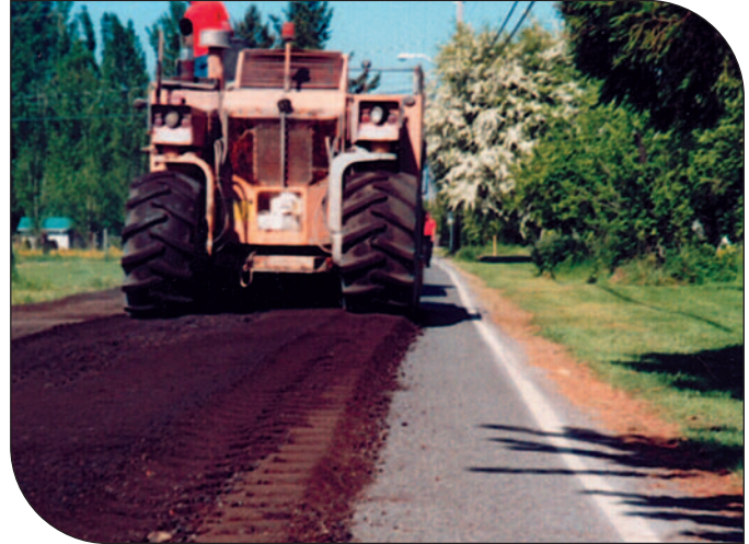
Pulverizing the old road.
